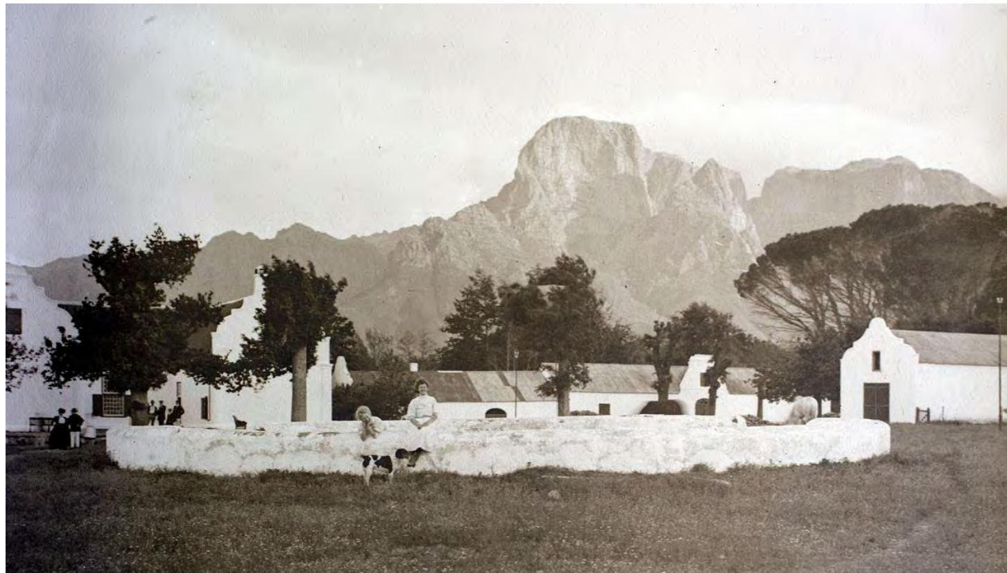
Figure 16: Boschendal werf in the late 19th early 20th century with threshing floor (foreground) and gabled wine cellar (centre) (Source: Boschendal Private Collection) The cellar has a corrugated iron roof, damaged central gable, two arched door openings and a single window.
