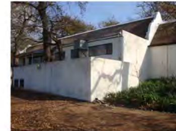
Existing service block to be converted.
