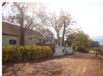
Existing service block to be converted.
