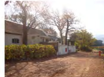
Existing service block to be converted.
