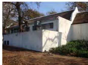
Existing service block to be converted.
