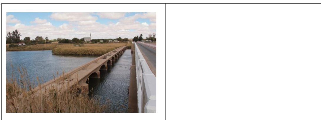
Fig. 9. Old bridge across the Orange River.
