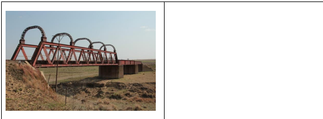
Fig. 20. The bridge across the Vaal River
