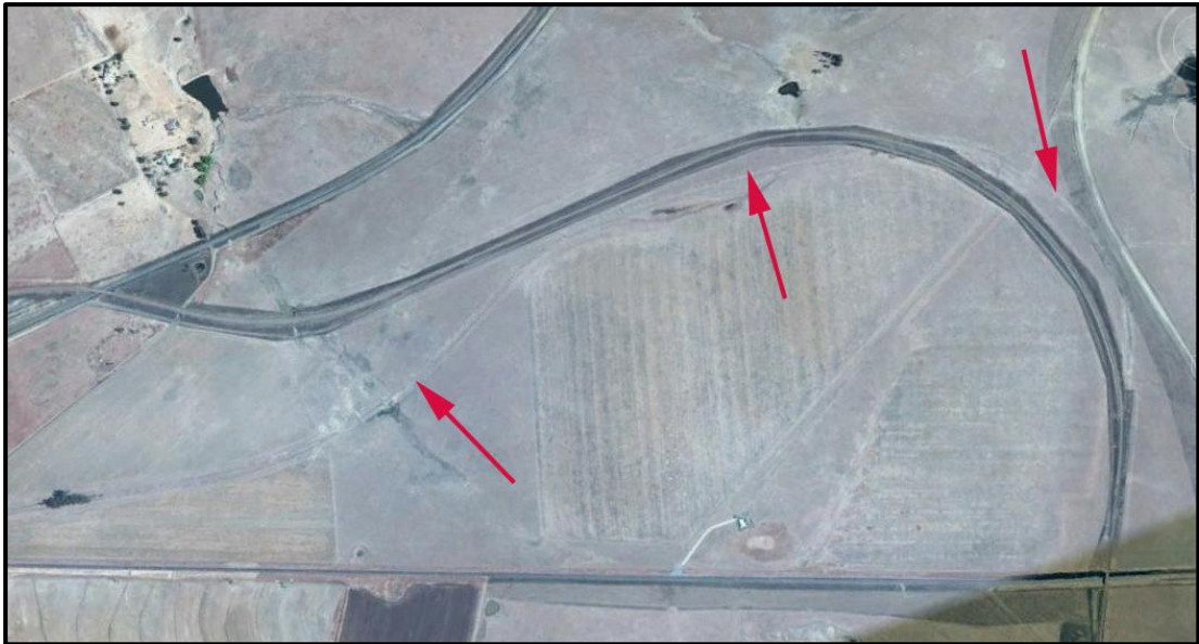
Fig. 12. A previous alignment of the railway line in the Davel region. (Photo: Google Earth)
