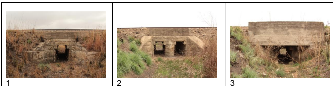
Fig. 16. Types of culverts on this section of the line.
