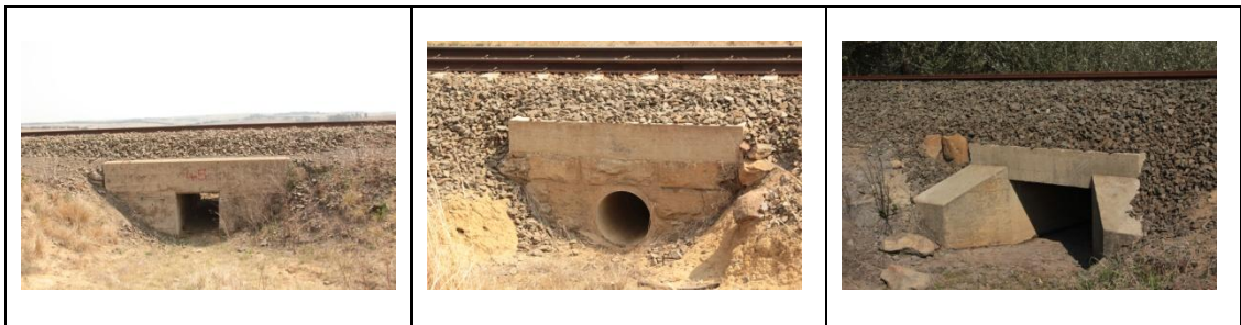
Fig. 18. Types of culverts on this section of the line.
