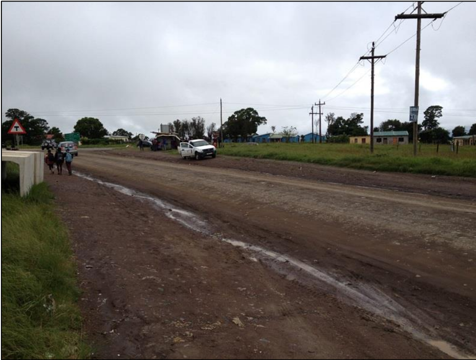
Figure 4-2: View of the southern offset of the Nkantolo road at the R61 intersection.
