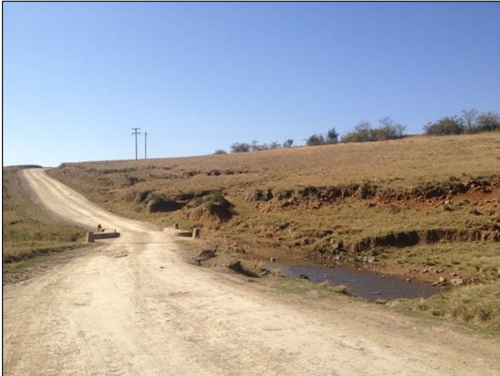
Figure 4-8: The Nkantolo access road where it transects the Ntlamvukazi River.
