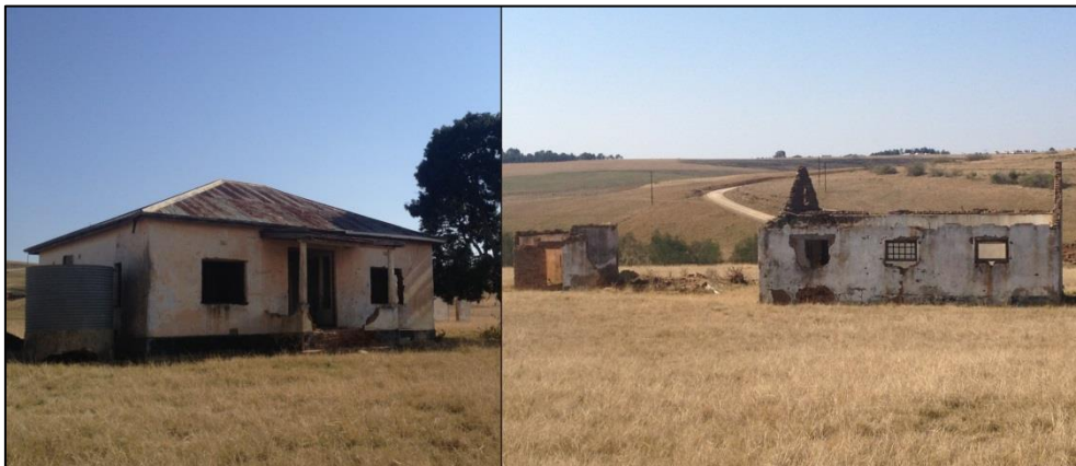
Figure 5-4: Deserted Western farmstead and outbuildings at Site HP02.
