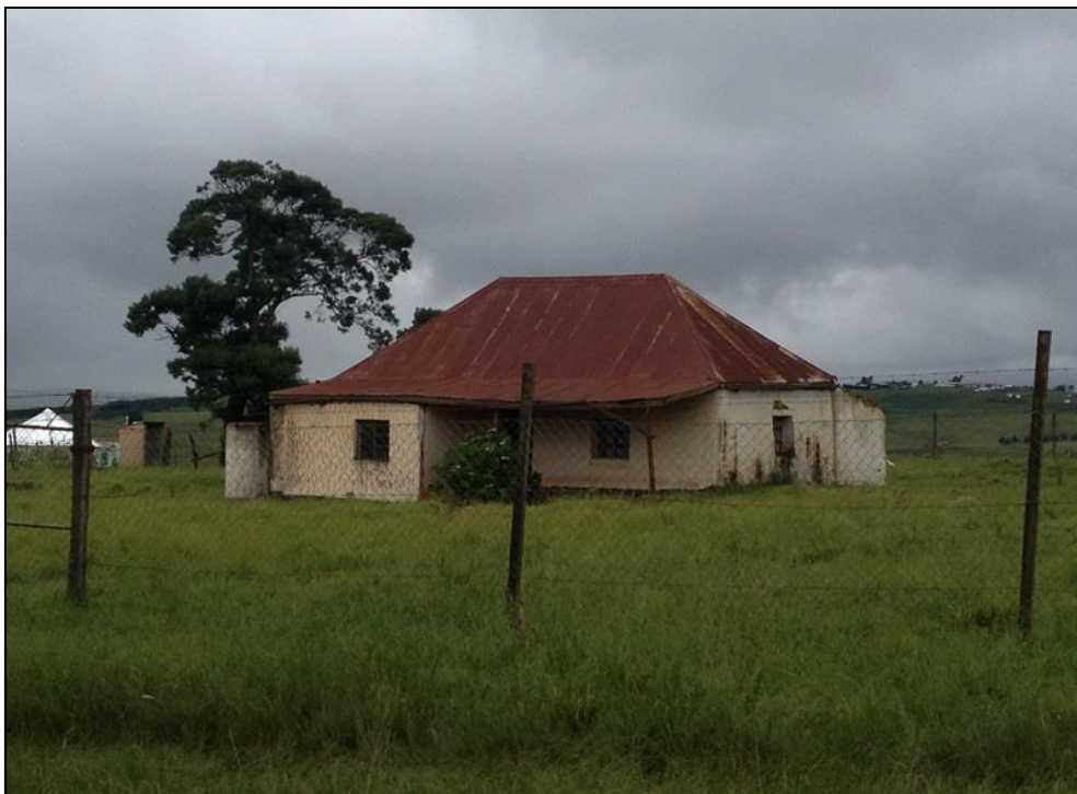
Figure 5-12: Western style building at site HP07.
