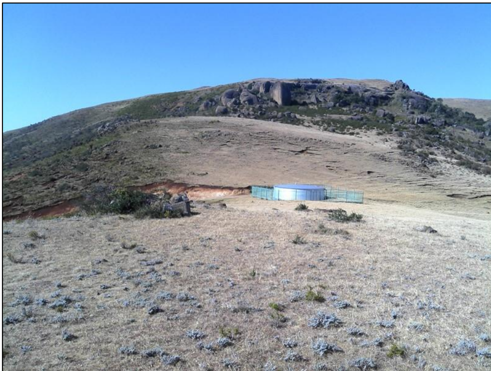
Figure 4-5: View of current reservoirs on a high ridge in the Emalawini area.
