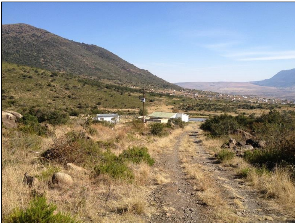
Figure 4-1: View of the current Mount Ayliff water treatments works east of the town.
