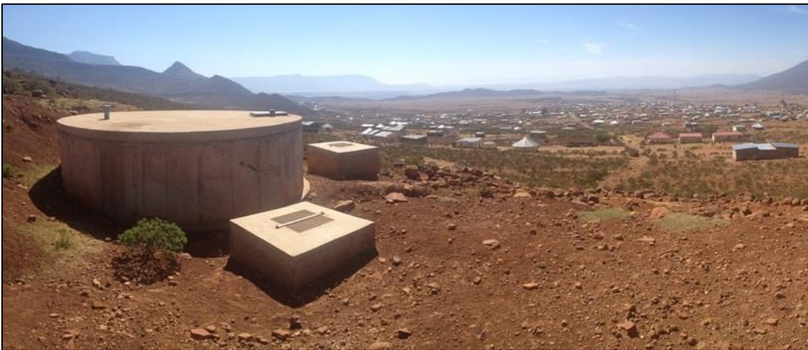
Figure 2-5: Existing reservoir and associated infrastructure on a ridge west of Noluthando.
