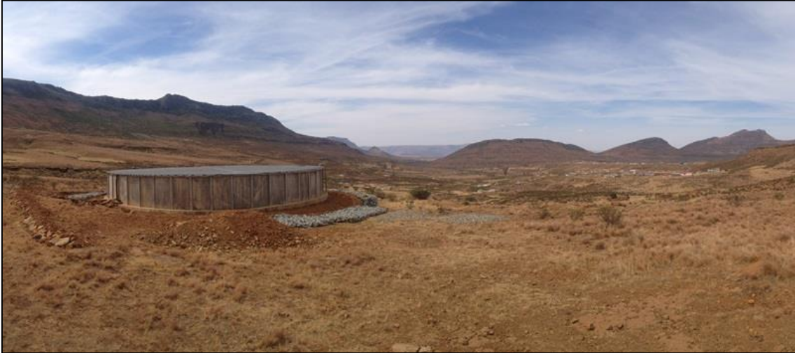
Figure 2-4: Existing reservoir on a high ridge south west of Lukhavala.
