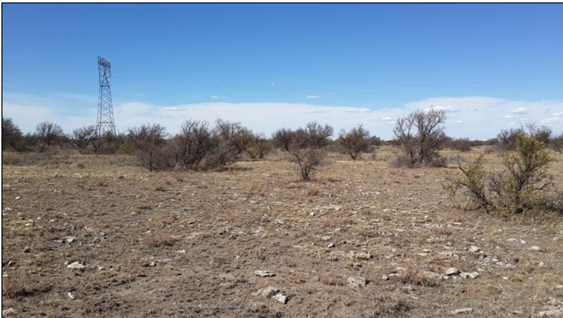
Figure 3-4: View of the northern periphery of the study area along the ESKOM power line.
