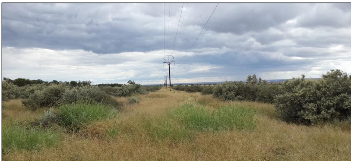
Figure 2-2: General surroundings on a portion of the farm Brandwagt along the footprint area for in the Carocraft Power Line at the time of the field survey (April 2014).
