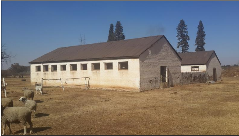
Figure 5-1: View of horse stables at Site Exigo-GD-HP01.
