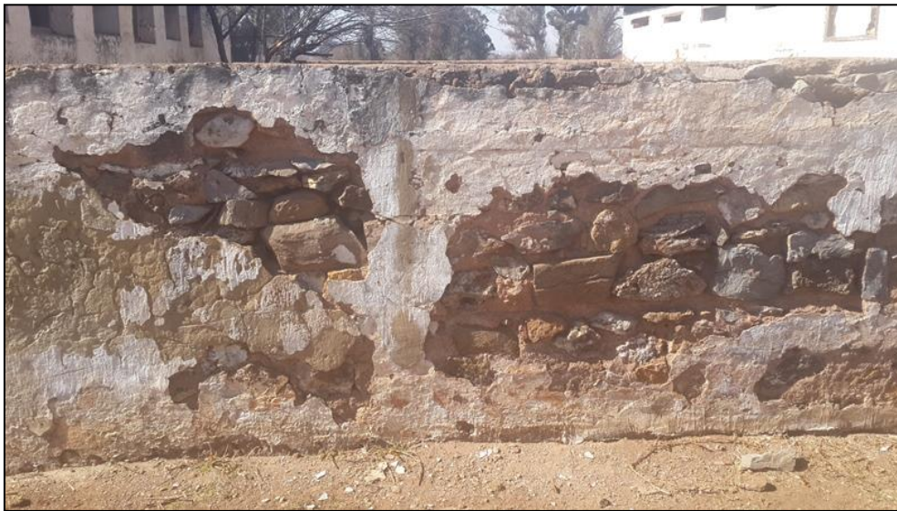
Figure 5-2: A section of stone wall at Site Exigo-GD-HP01. Note the use of mud clay as cement in the construction.
