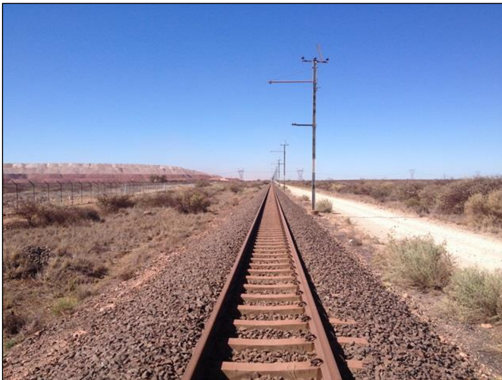
Figure 3-1: View of the existing Transnet railway line at the site of the proposed HEF rail link connection.
