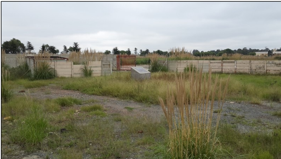
Figure 3-7: A walled area indicating the presence of subterranean power lines to the west of the project area.
