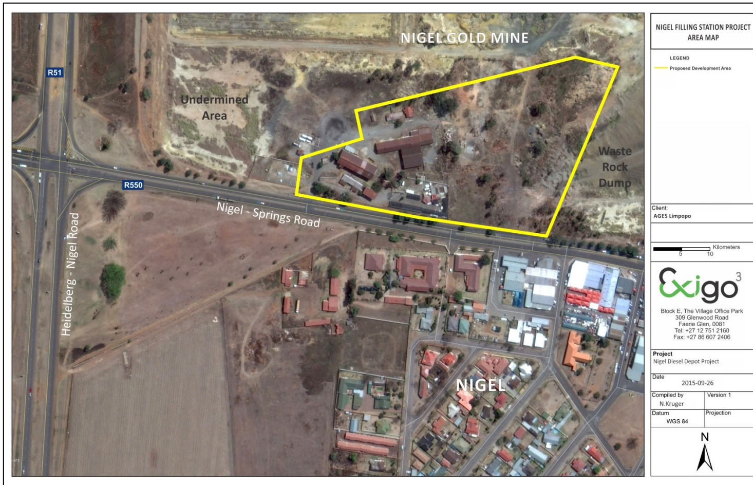
Figure 2-2: Aerial representation of the regional setting for the Nigel Diesel Depot Project area.
