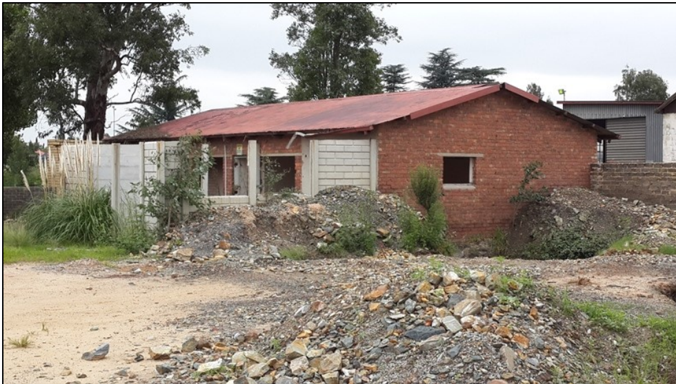
Figure 5-8: A deserted red face brick structure Site EXIGO-VF169-FT04.
