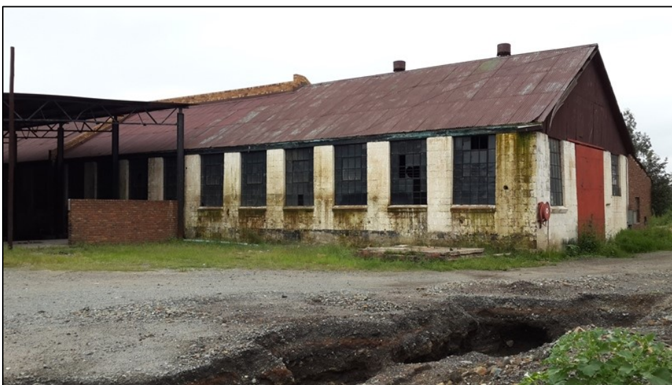
Figure 5-4: A warehouse building at Site EXIGO-VF169-HP03.
