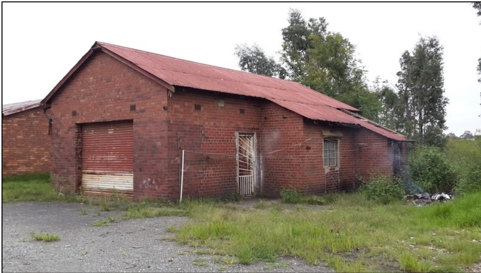
Figure 5-2: A small Colonial Period face brick building at Site EXIGO-VF169-HP01.
