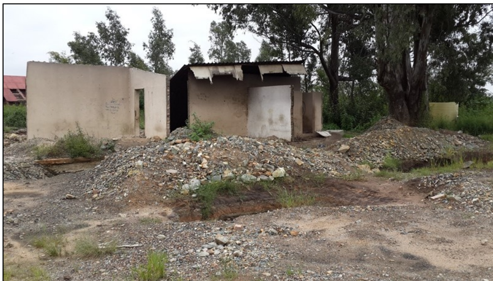
Figure 5-11: Dilapidated structures and foundations at Site EXIGO-VF169-FT05
