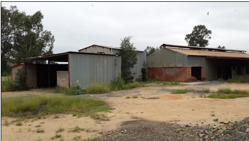
Figure 3-1: View of existing structures in the project area.
