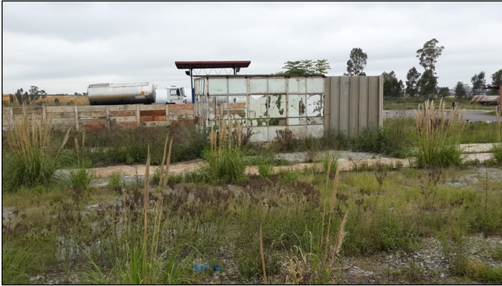
Figure 3-6: An existing small fuel depot in the project area.
