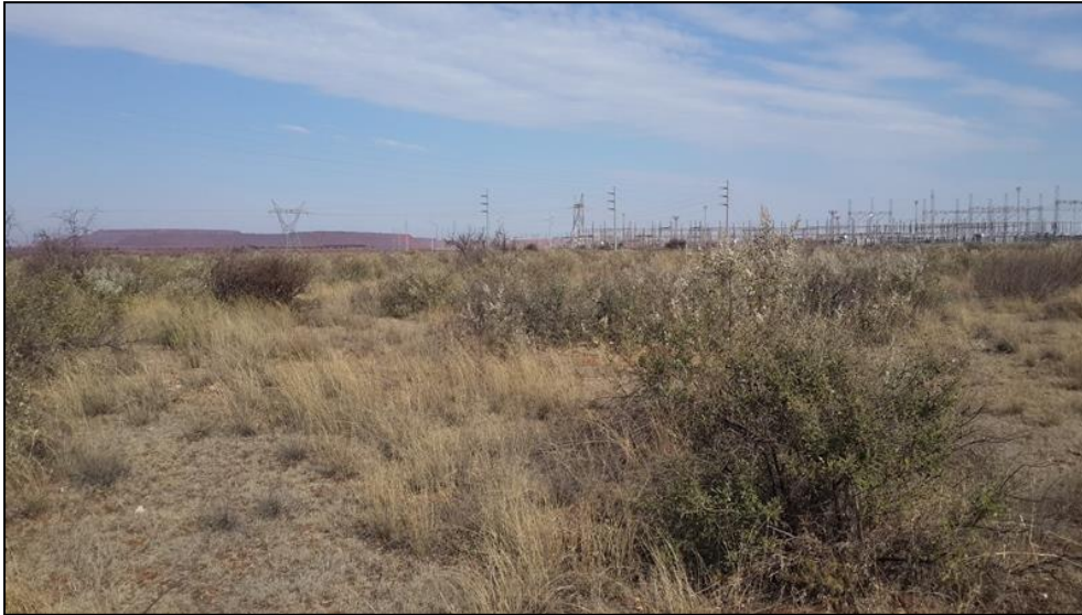
Figure 3-1: View of general surroundings at the existing Ferrum substation, looking west.
