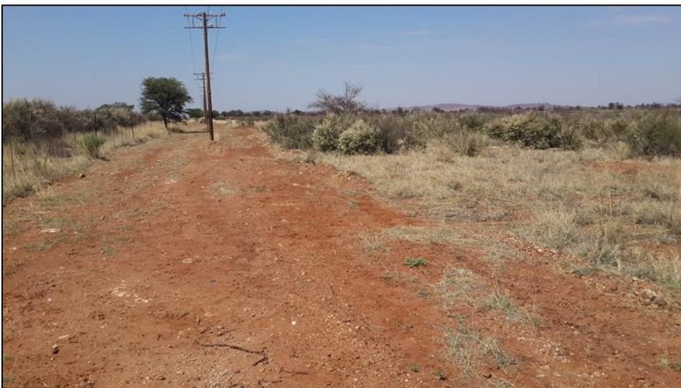
Figure 3-8: The eastern boundary of the proposed Sekgame switching yard site next to the N14 National road.
