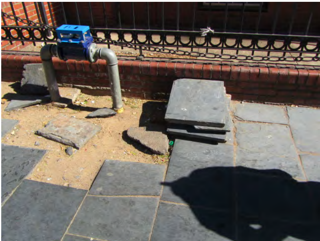
Fig. 110 Smaller sections of flagstone are used around fixtures. (Photograph SM Miller 2012)
