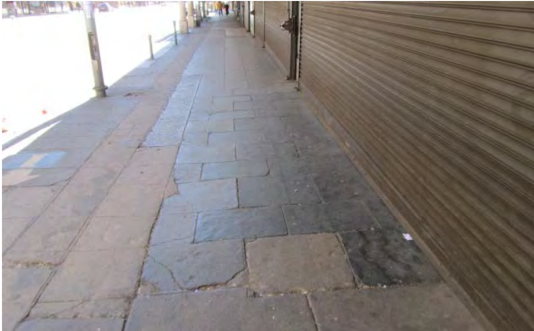
Figure 8 Remains of historical slate flagstone on the eastern side of Block 5. (Photograph SM Miller 2012)
