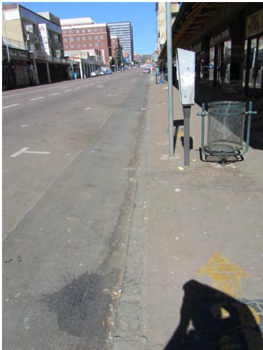
Figs 78 and 79 Above left is the granite kerbing on the north-western side of Block 5. Above right are the vehicular access areas for PGC-HOUSE where the granite kerbing was not removed but lowered for access. (Photographs SM Miller 2012)
