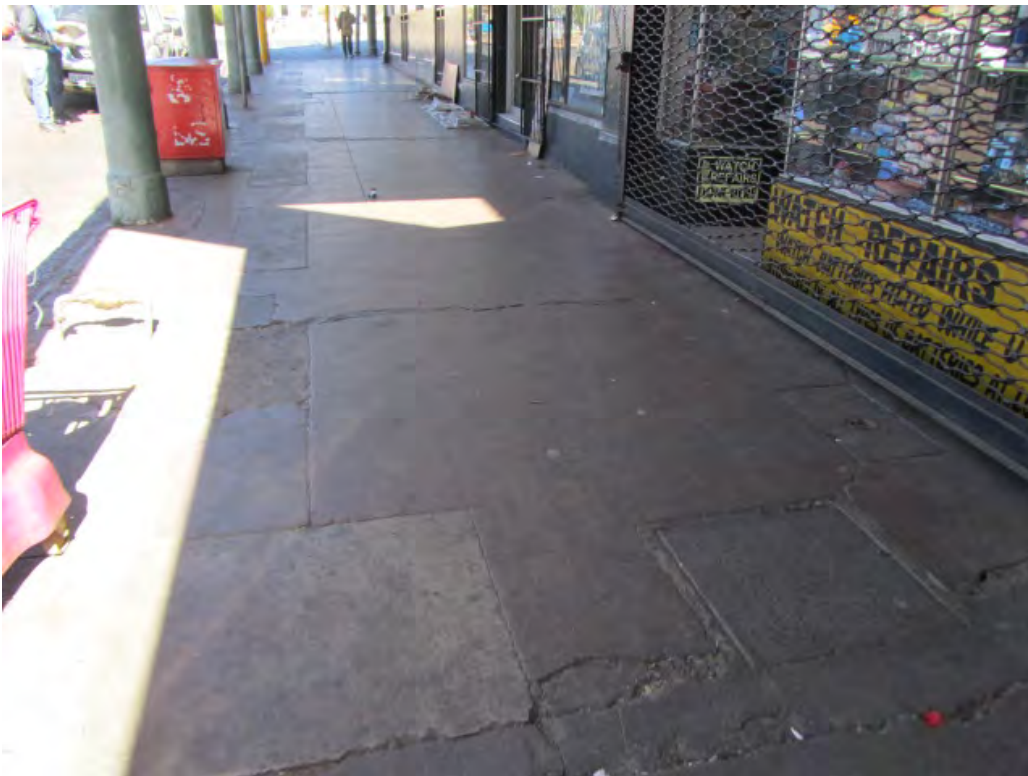
Fig. 166 Another view of the canopy support columns of the old Victoria Hotel. Note replacement of the slate flagstones with ferro-granolite concrete panels. (Photograph SM Miller 2012)
