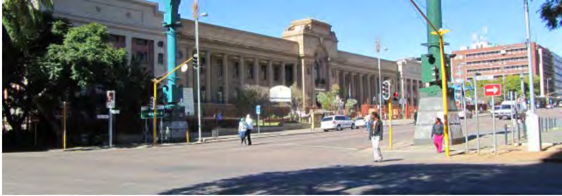
Fig. 123 Block 8, which includes the Old Town Hall, contains the largest section of in situ slate flagstones. This area will have to feature in proposal on preservation and also the design of new elements. (Photograph SM Miller 2012)
