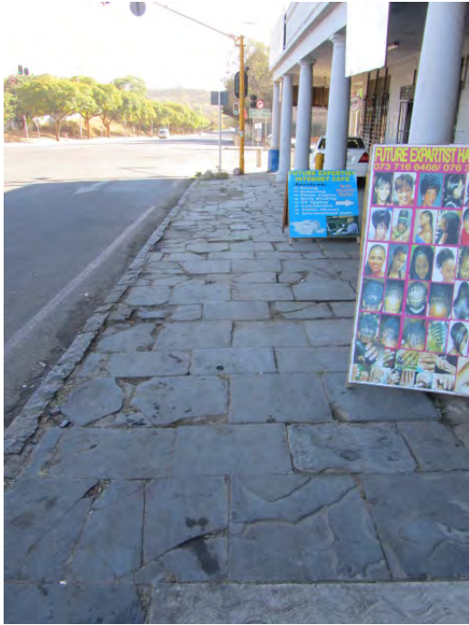
Figs 6 and 7 Historical slate flagstones, granite kerbing and pillars of sidewalk in front of protected building. (Photographs SM Miller 2012)
