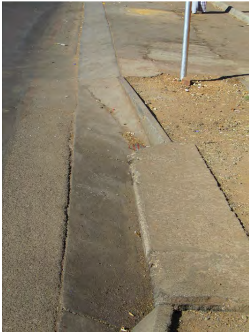
Figs 36 and 37 Kerbing along the northern and southern ends of the western sidewalk in Block 2. A section of the sidewalk has been forfeited for parking and a 50 meter section of granite kerbing was removed. Three vehicular access points exist in the northern section. (Photographs SM Miller 2012)
