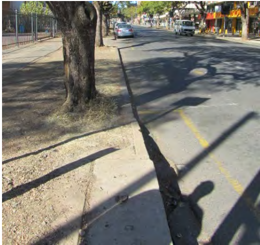
Figs 48 and 49 Location of historical granite kerbing on both the north-eastern and north-western ends of Block 3. Concrete strips are the main paving products on both sidewalks. (Photographs SM Miller 2012)
