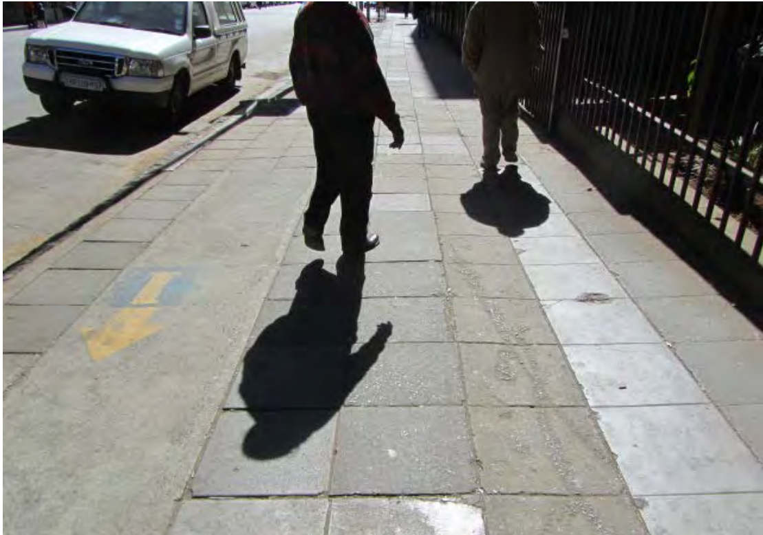
Fig. 93 View of granite kerbing. Note complete absence of slate flagstones. (Photograph SM Miller 2012)
