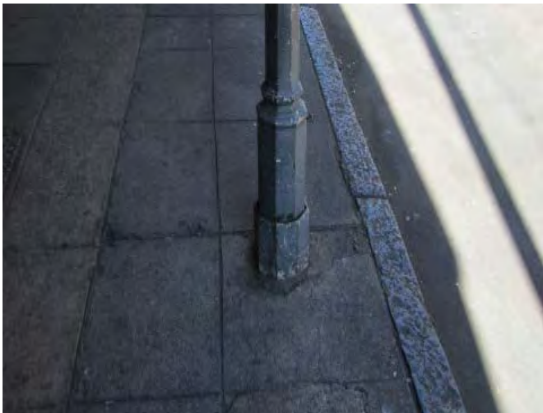
Figure 8 Only a few of these Edwardian shop veranda cast iron column bases remain on Paul Kruger Street. It is important that they are retained. (Photograph SM Miller 2012)
