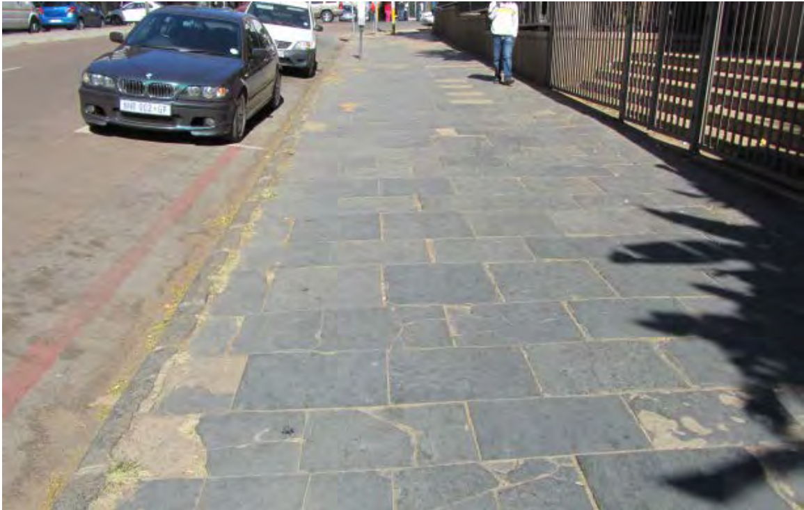
Fig. 153 Another view of the south-western part of Block 9 where most of the original slate flagstone paving blocks remain. As elsewhere in the study area the paving is in a poor state of repair. Note variation in the placement of different types of flagstones. (Photograph SM Miller 2012)
