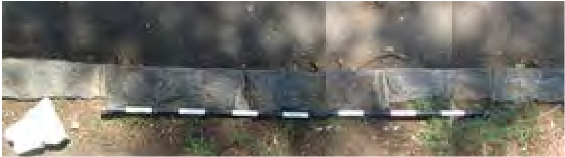
Fig. 62 Length of the granite kerbing on the west side of Block 3, being from 300 to 500 mm (12 and 20 inches). This may vary as the kerb stones were handmade. (Photograph SM Miller 2013)
