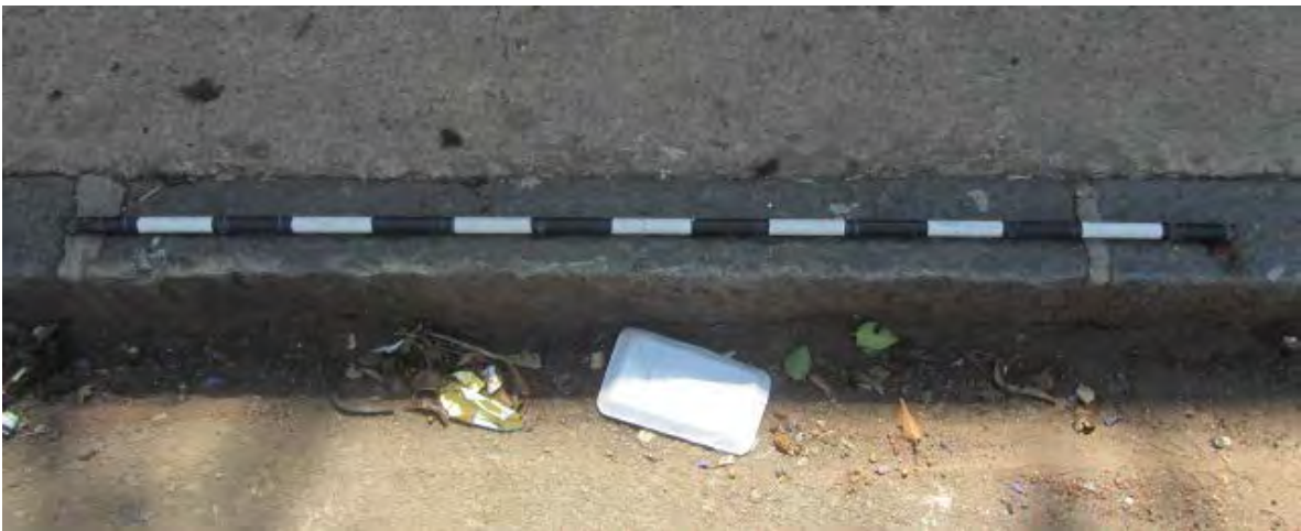
Fig. 63 In some areas the granite kerbing is even more variable up to a length of 1300 mm (four foot six inches). (Photograph SM Miller 2013)
