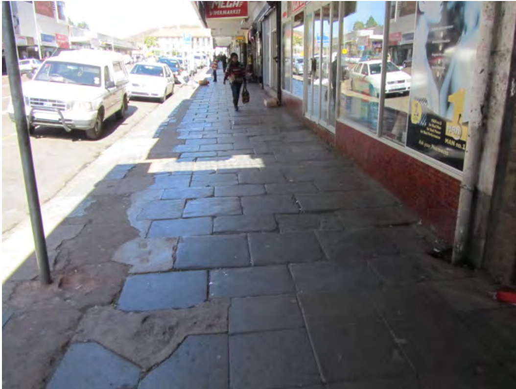
Fig. 163 Slate flagstone paving in the central western side of Block 10. Note the impact of placement of services. (Photograph SM Miller 2012)
