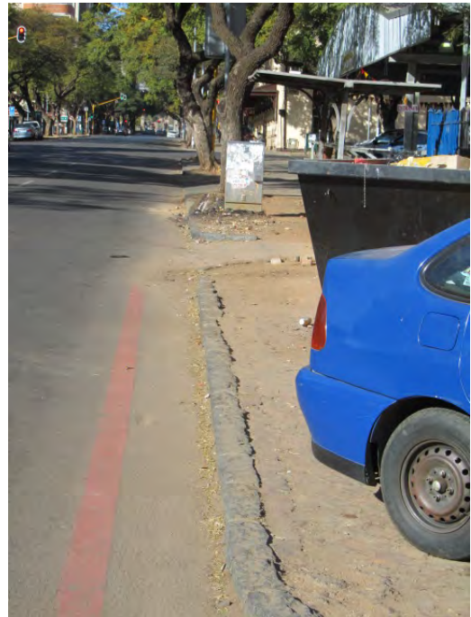
Figs 36 and 37 Kerbing along the northern and southern ends of the western sidewalk in Block 2. A section of the sidewalk has been forfeited for parking and a 50 meter section of granite kerbing was removed. Three vehicular access points exist in the northern section. (Photographs SM Miller 2012)
