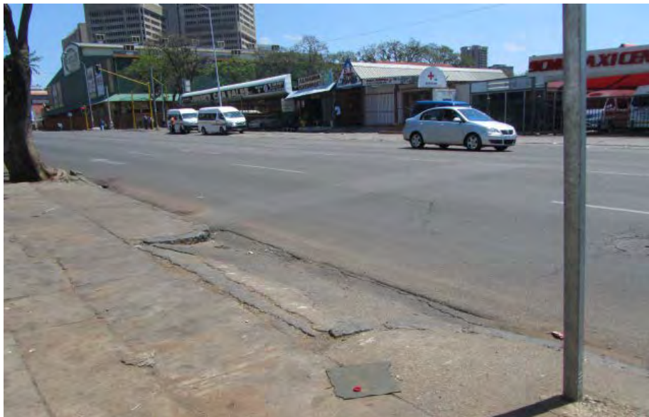
Fig. 21 Intervention for vehicular access to previous dwellings and existing businesses such as depicted above occurs along the eastern side of Paul Kruger Street. These vary from three to nearly 5 meters (Photograph SM Miller 2013)
