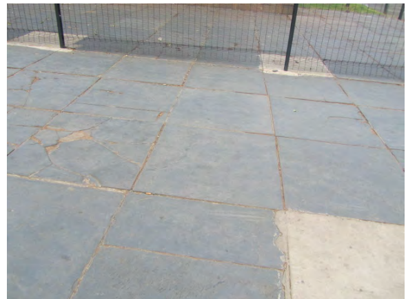
Figs 125 and 126 Left is an example where inappropriate material that is not compatible with the historical features has been used. The installation of storm water drainage that necessitated culverts resulted in this unfortunate solution. Above right we see the impact of the installation of a security fence on the historical flagstone paving. (Photograph SM Miller 2013)
