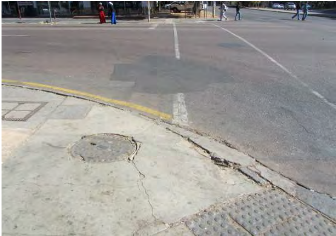
Fig. 105 In most cases wheelchair access were facilitated without the removal of historical granite kerb stones. (Photograph SM Miller 2012)
