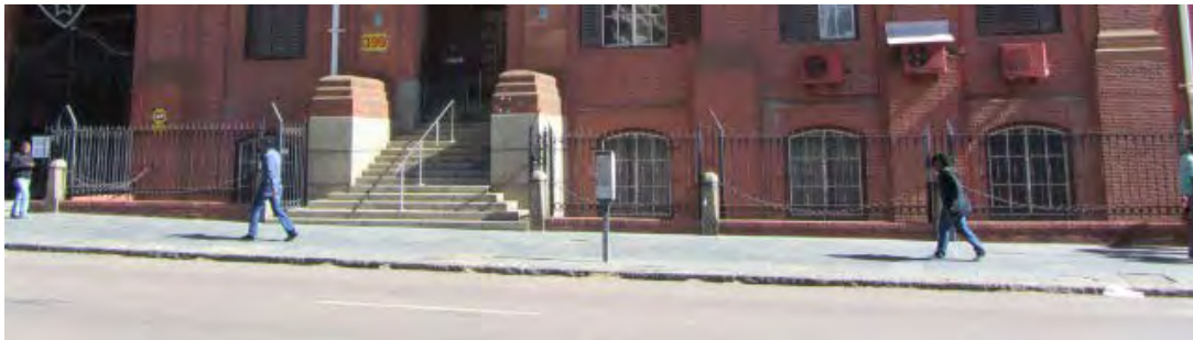
Fig. 102 A record of historical granite kerb stones as well as slate flagstones. (Photograph SM Miller 2012)
