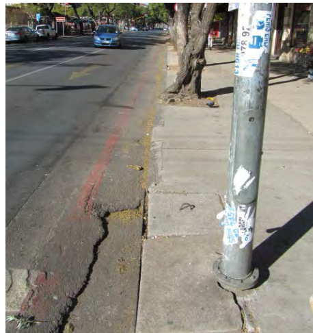
Figs 48 and 49 Location of historical granite kerbing on both the north-eastern and north-western ends of Block 3. Concrete strips are the main paving products on both sidewalks. (Photographs SM Miller 2012)
