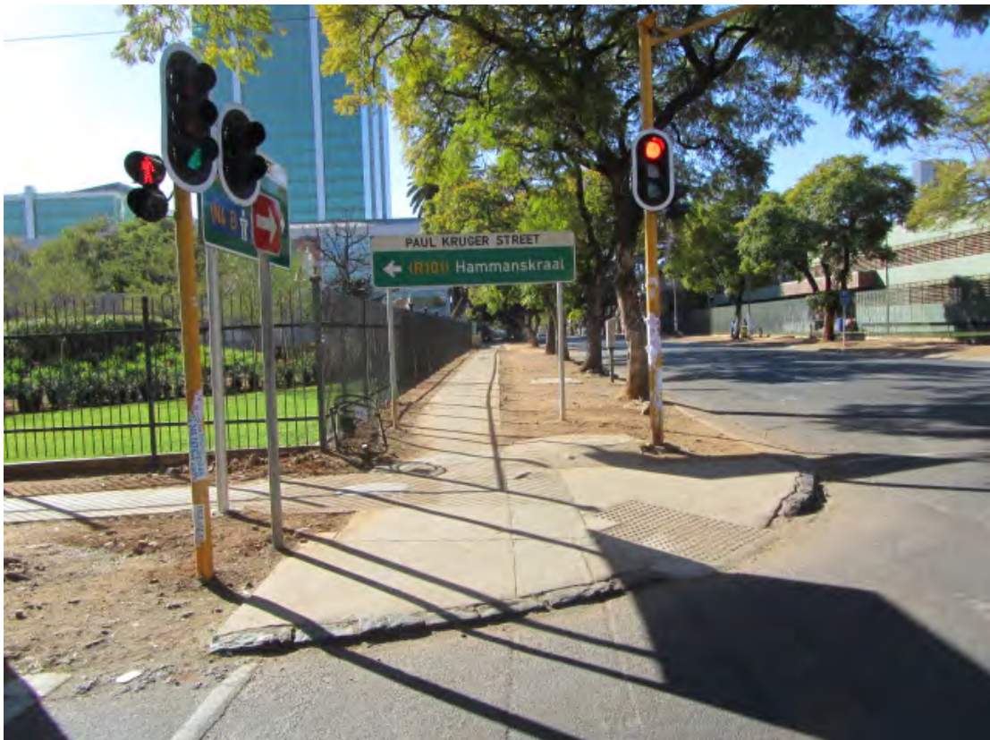
Fig. 40 Granite kerbing was adapted throughout the study area at street corners to accommodate physically-disadvantaged people. In some cases granite kerb stones were retained, while at other places modern materials were used. (Photograph SM Miller 2012)
