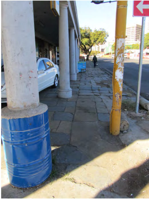
Figs 9 and 10 Historical slate flagstones on the sidewalk in front of protected building and granite kerbing on eastern side of Paul Kruger Street in Block 1. (Photographs SM Miller 2012)
