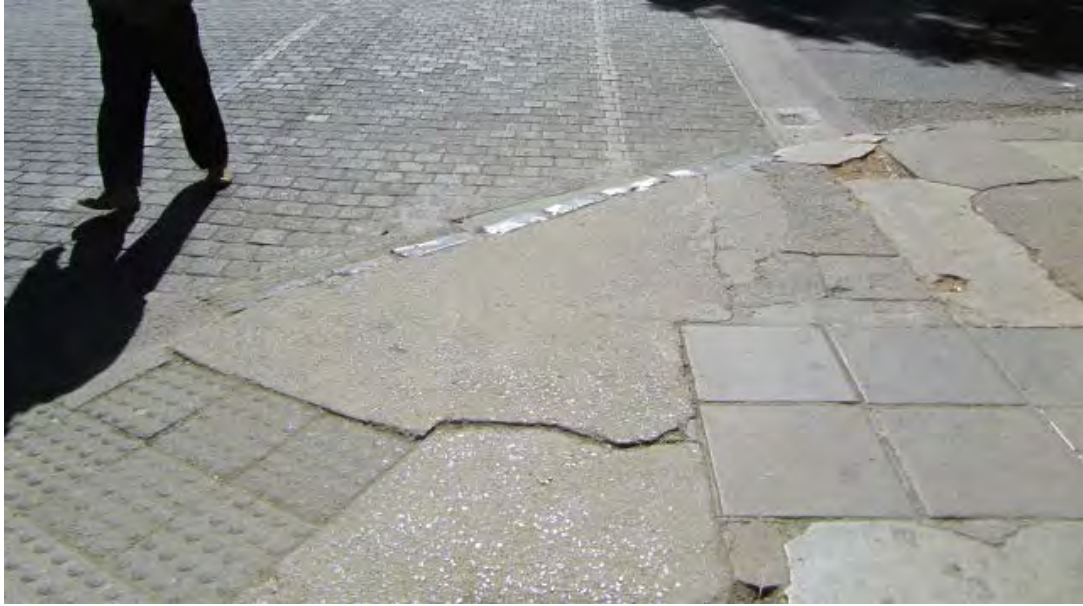
Fig. 146 New road paving as part of the Museum walk renovation several years ago. Sidewalk paving is neither aesthetically pleasing, nor is it safe for pedestrians.. (Photograph SM Miller 2012)
