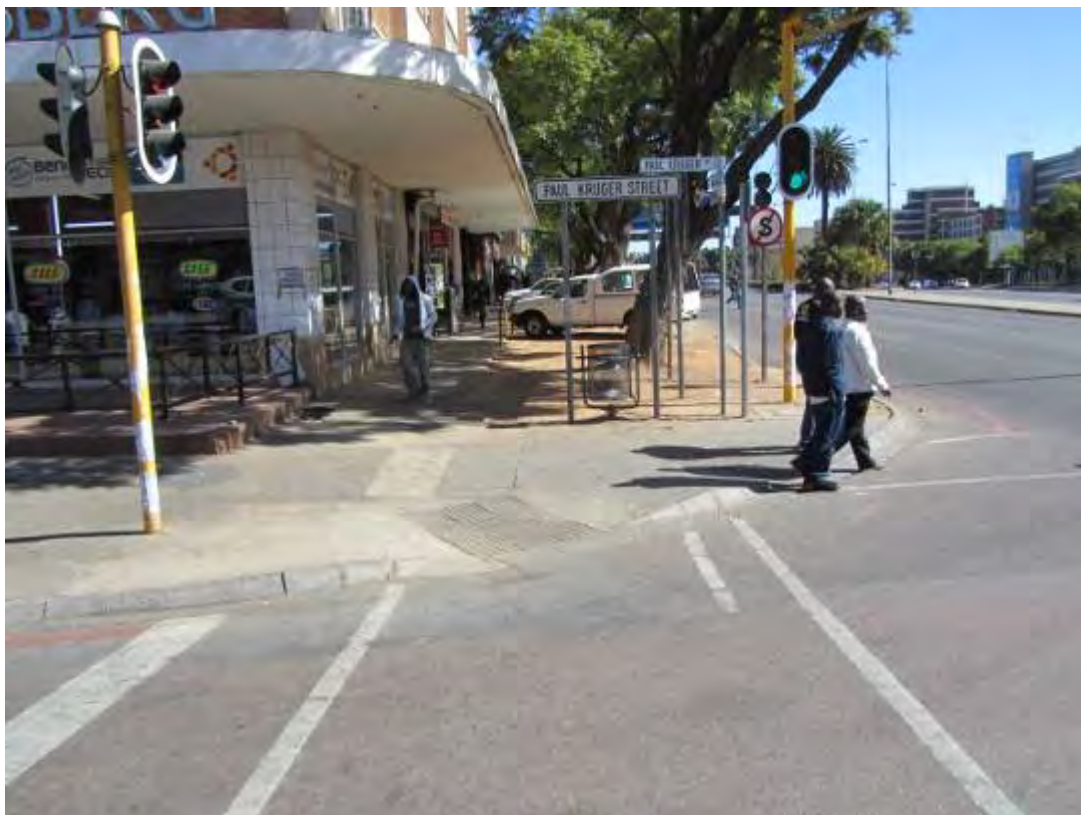
Fig. 106 At several locations new kerbing was installed during provision of wheelchair accessibility. (Photograph SM Miller 2012)
