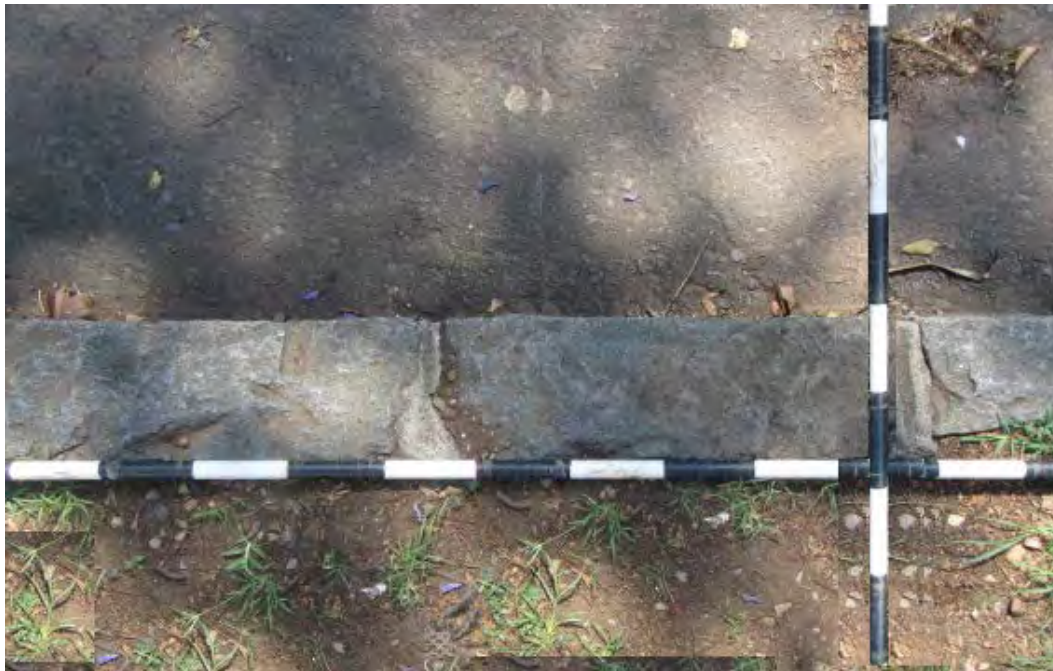
Fig. 61 Width of granite kerbing on the west side of Block 3 of between 150 to 200 mm (6 and 8 inches.) This may vary as the kerb stones were handmade. (Photograph SM Miller 2013)
