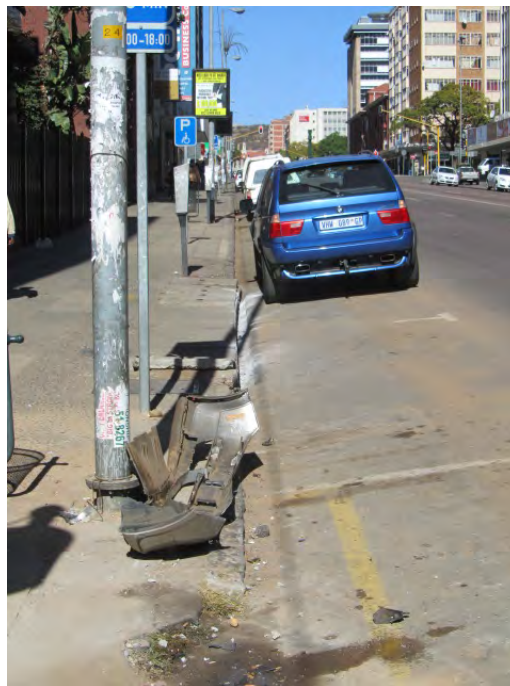
Figs 91 and 92 Two views along granite kerbing. Note complete absence of slate flagstones. (Photographs SM Miller 2012)
