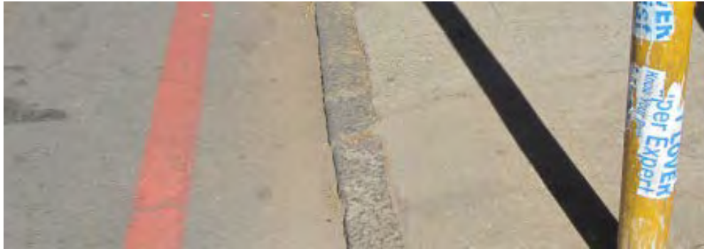
Fig. 149 The image above captures a typical situation in the city where the level of granite kerbing is impacted upon by continuous road re-surfacing. (Photograph SM Miller 2012)
