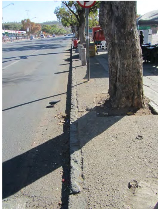
Figs 9 and 10 Historical slate flagstones on the sidewalk in front of protected building and granite kerbing on eastern side of Paul Kruger Street in Block 1. (Photographs SM Miller 2012)
