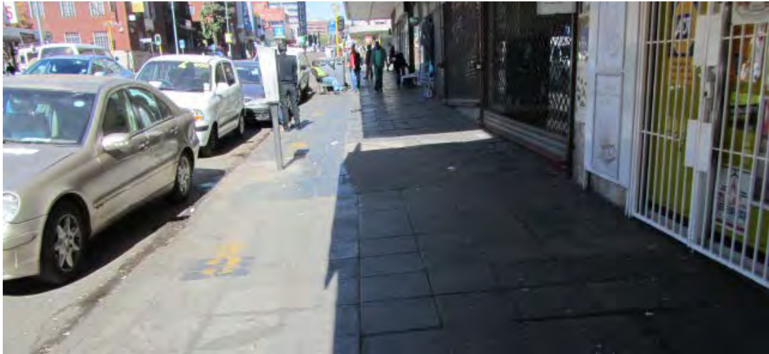
Fig. 80 Granite kerbing on the north-western side of Block 5. In the centre of the image are random remaining slate flagstones. (Photograph SM Miller 2012)
