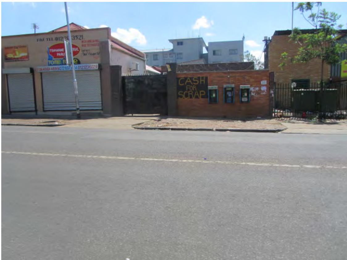
Figs 43 Granite kerbing on the west side of Block 2 and vehicular access areas for the building in the background. (Photograph SM Miller 2013)
