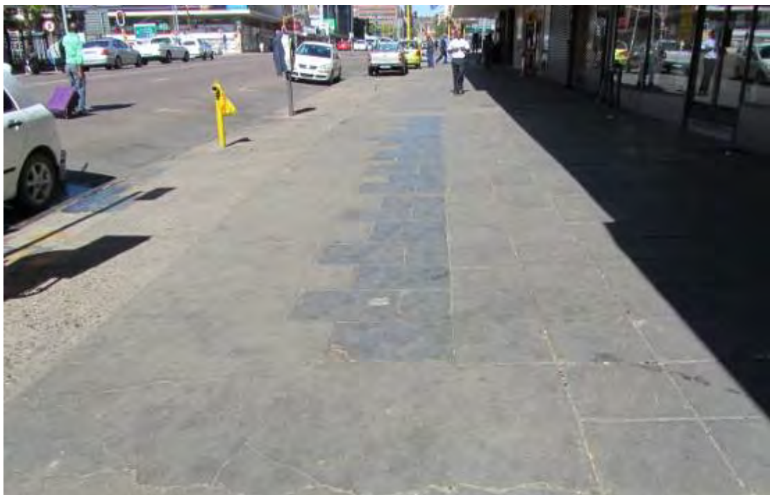
Fig. 94 A variety of paving material on the western side of Paul Kruger Street in Block 6. Remnants of slate flagstone paving are also visible. (Photograph SM Miller 2012)
