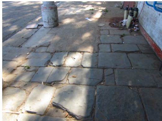
Figs 9 and 10 Historical slate flagstones on the sidewalk in front of protected building and granite kerbing on eastern side of Paul Kruger Street in Block 1. (Photographs SM Miller 2012)
