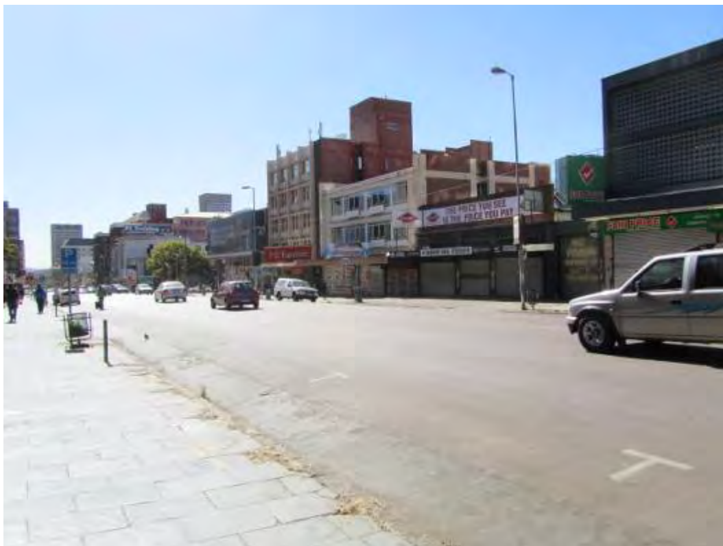
Fig. 112 Record of slate flagstone paving on the south-western corner of Paul Kruger and Visagie streets. ( Photograph SM Miller 2012 )
