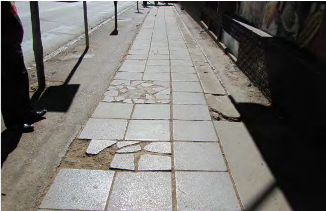
Fig. 154 On the eastern side of Block 9 only the granite kerb stones remain. All slate flagstones have been removed and replaced with modern materials. (Photograph SM Miller 2012)
