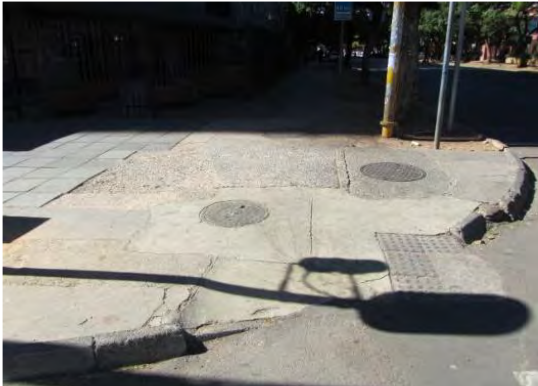
Fig. 114 Note wheelchair access on the south-eastern corner of Block 7. (Photograph SM Miller 2012)
