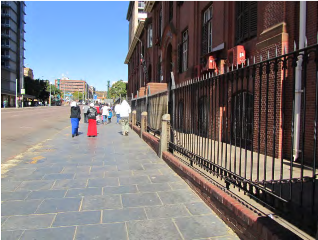
Fig. 109 A record of yet another section of slate flagstone paving on the western side of Block 7. Note style of alternating square blocks with rectangular ones. (Photograph SM Miller 2012)
