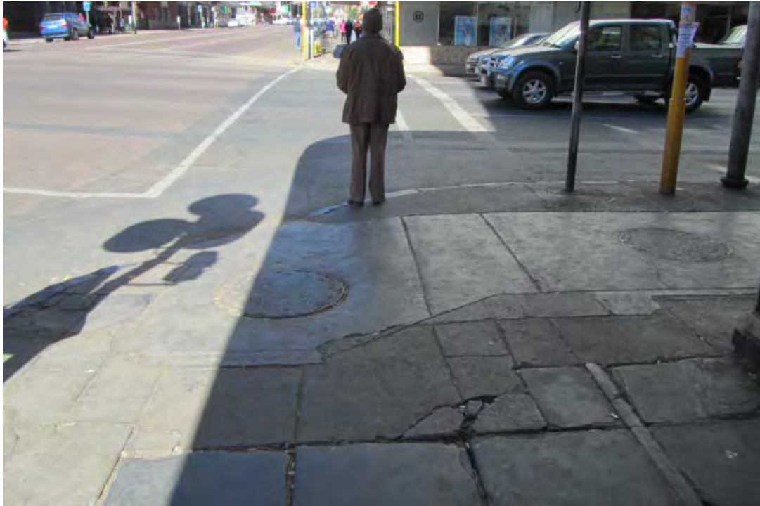
Fig. 82 Southwest corner of Block 5 where historical granite kerbing was retained but adjusted to a lower level to enable wheelchair access. This is apparent at most corner localities. (Photograph SM Miller 2012)
