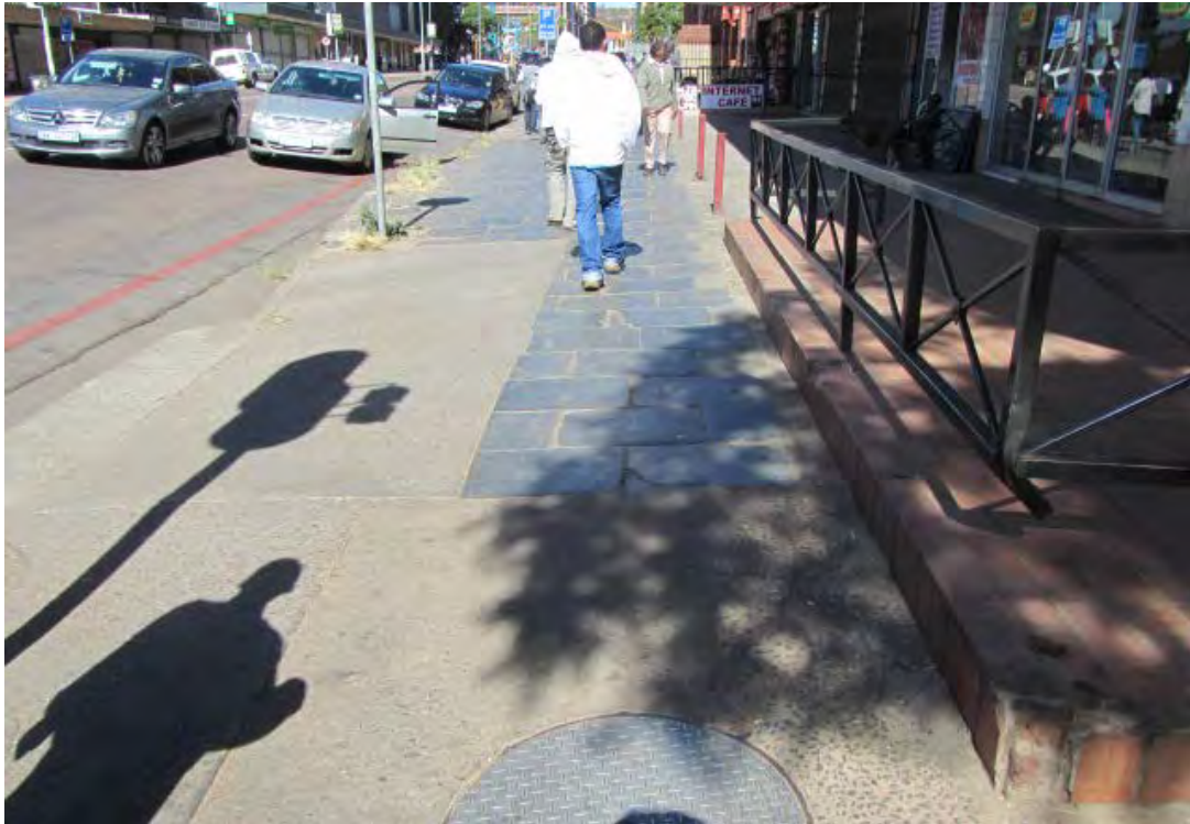
Fig. 107 On the western side of Block 7 a particularly large section of slate flagstone paving survives. It may be on account of the smaller rectangular format of the flagstones that have been used. (Photograph SM Miller 2012)
