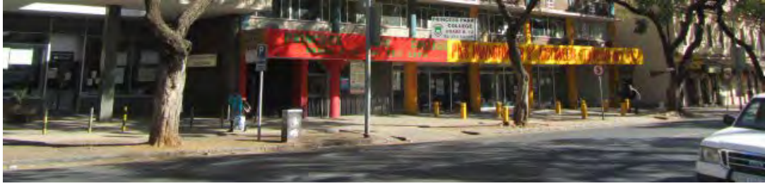
Fig. 57 Granite kerbing defining old roadway and vehicular access on both sides of red- and yellow-painted building. (Photographs SM Miller 2012)
