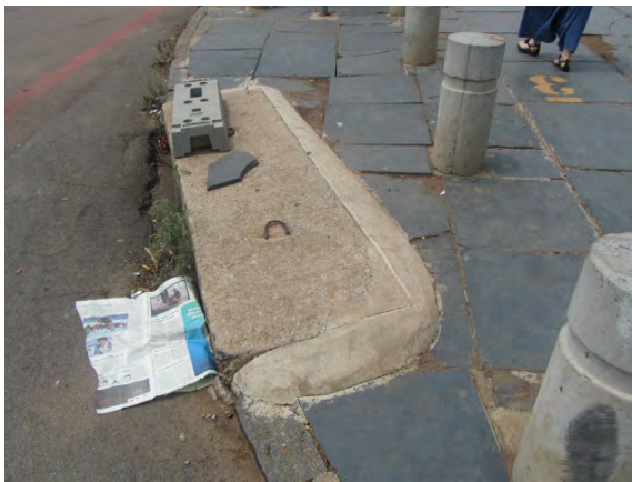
Figs 125 and 126 Left is an example where inappropriate material that is not compatible with the historical features has been used. The installation of storm water drainage that necessitated culverts resulted in this unfortunate solution. Above right we see the impact of the installation of a security fence on the historical flagstone paving. (Photograph SM Miller 2013)
