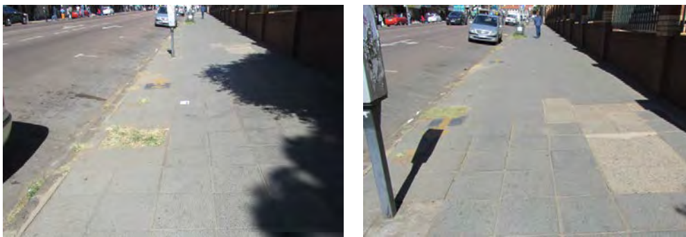
Figs 150 and 151 In this location the slate flagstones were replaced with modern paving blocks. It appears as if some attempt was made to imitate the colour of the flagstones as these blocks have a blue tinge. (Photograph SM Miller 2012)
