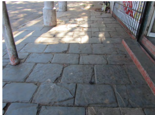
Figs 9 and 10 Historical slate flagstones on the sidewalk in front of protected building and granite kerbing on eastern side of Paul Kruger Street in Block 1. (Photographs SM Miller 2012)
