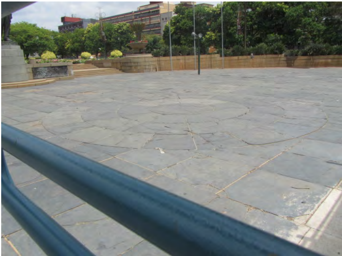
Fig. 134 This is the only decorative pattern in areas that retain slate flagstone paving. Unfortunately a security gate does not allow access into the paved area in front of the Town Hall. (Photograph SM Miller 2013)
