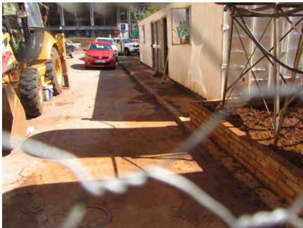
Fig. 42 Contractor's site office in Mutual Street. (Photograph SM Miller 2013)
