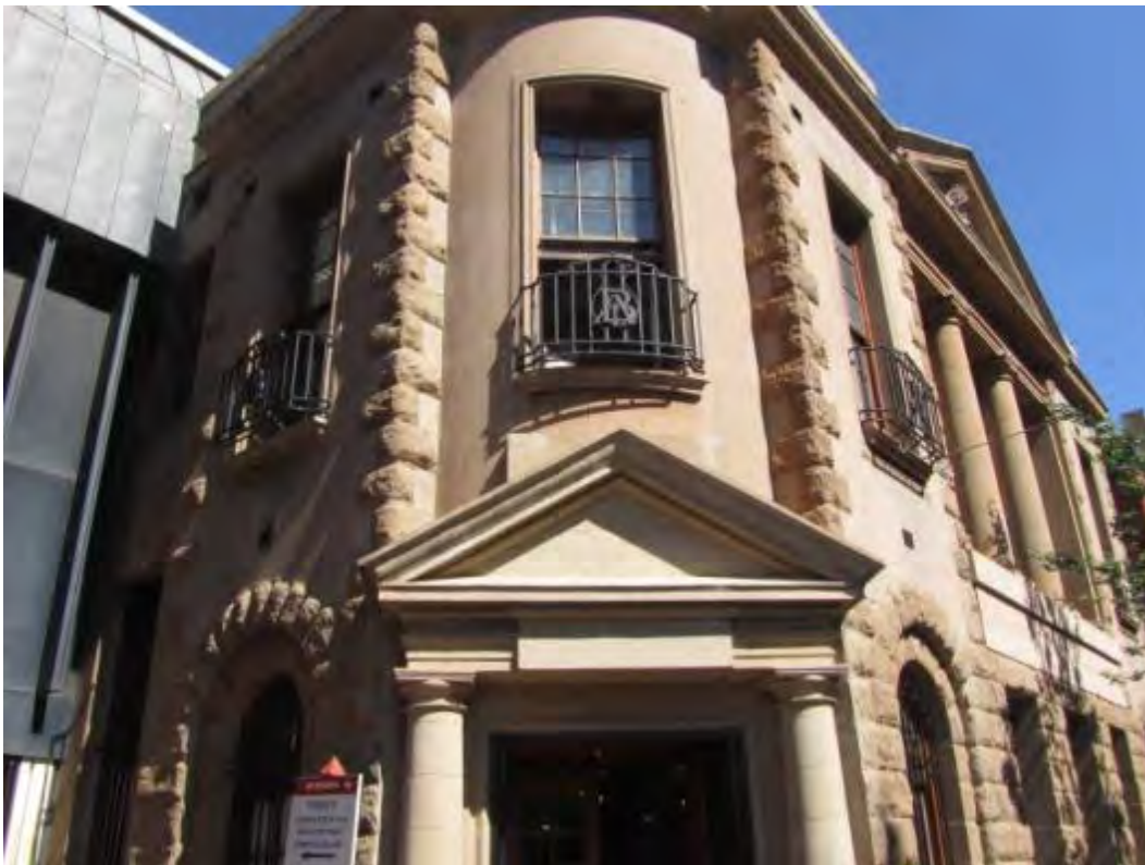
Fig. 29 Detail of protected building. (Photograph SM Miller 2013)
