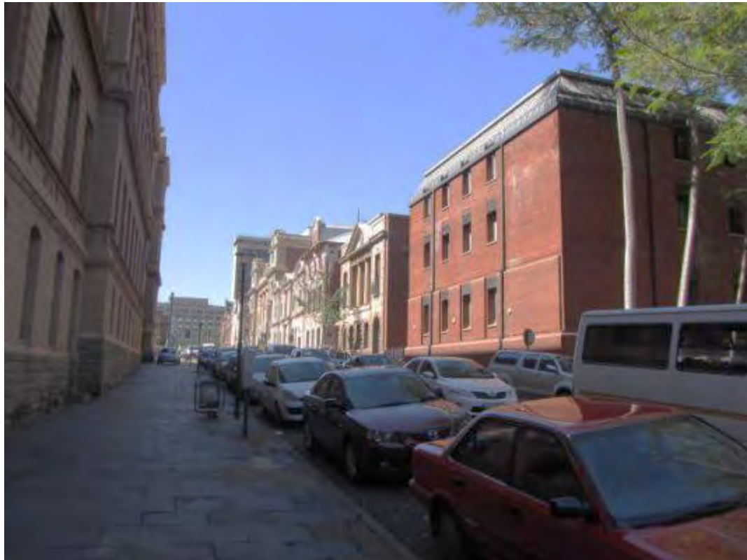
Fig. 24 Historical slate flagstone paving and historical granite kerbing along the north-eastern section of Block 1. (Photograph SM Miller 2013)
