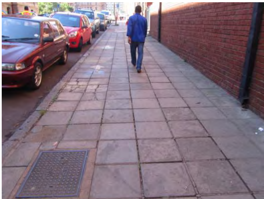
Fig. 27 Modern paving and historical granite kerbing along the central western section of Block 1. (Photograph SM Miller 2013)
