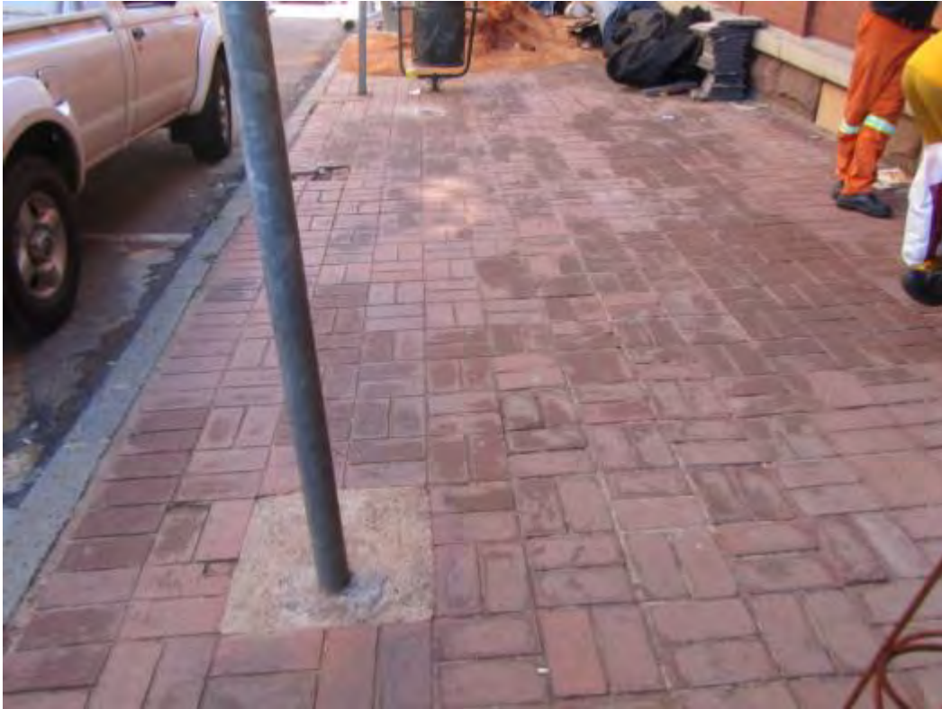
Fig. 34 Modern paving and historical granite kerbing along the south-eastern section of Block 2. (Photograph SM Miller 2013)
