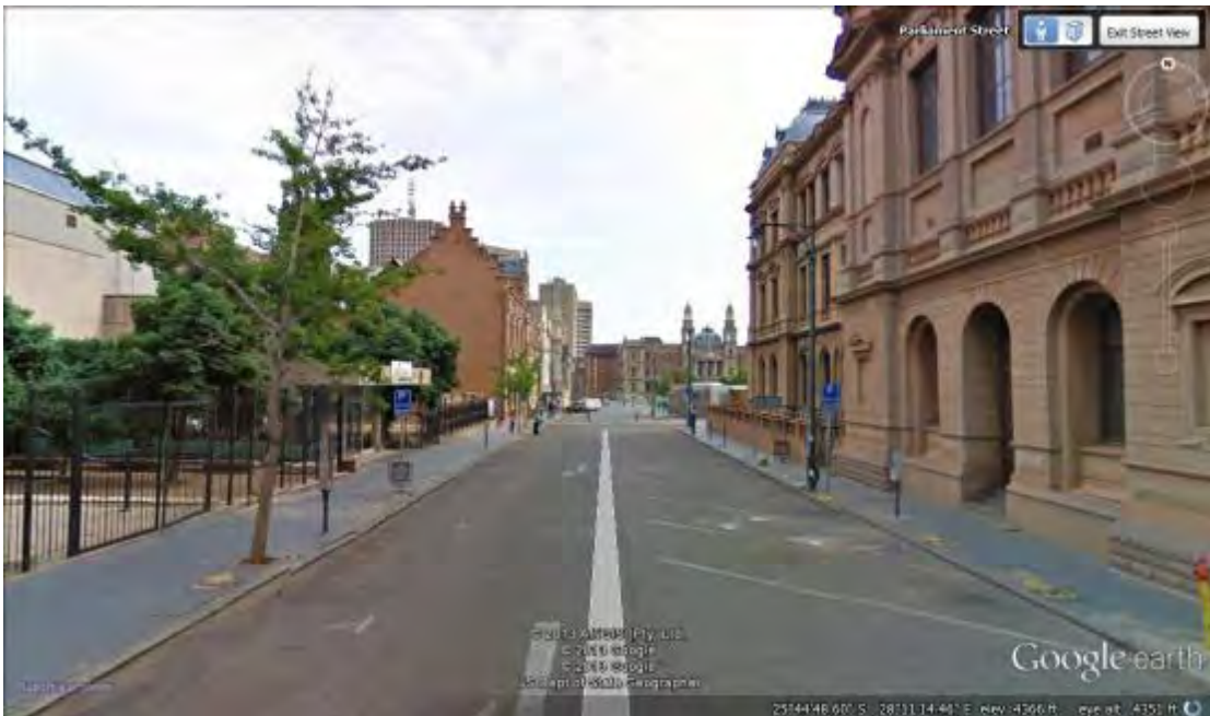
Fig. 59 This image from 2009 provides a view of the actual conditions in Mutual Street regarding paving and granite kerbing. (Google Earth Street view 2009)
