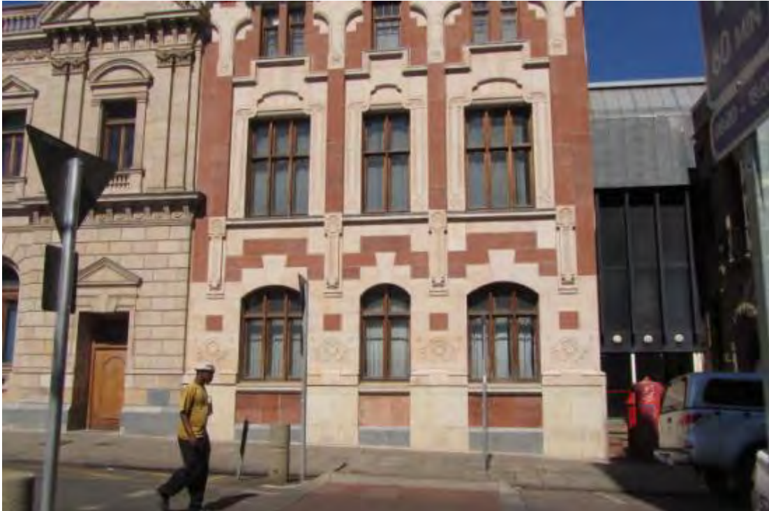
Fig. 20 A record of a protected building (National Bank and Mint 1892). Note historical granite kerbing but absence of slate flagstone paving at the south end of Palace Street. (Photograph SM Miller 2013)
