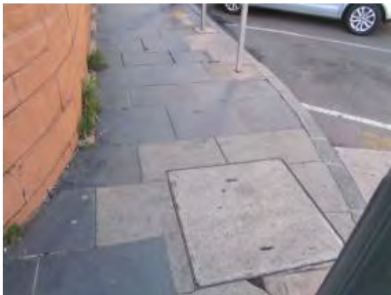
Figs 52 and 53 Historical slate flagstone paving and historical granite kerbing along the north-eastern section of Block 3. (Photograph SM Miller 2013
