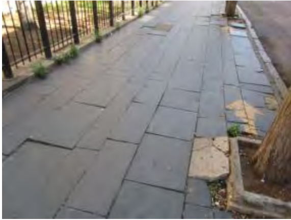
Figs 48 and 49 Historical slate flagstone paving and historical granite kerbing along the south-western section of Block 3. (Photograph SM Miller 2013
