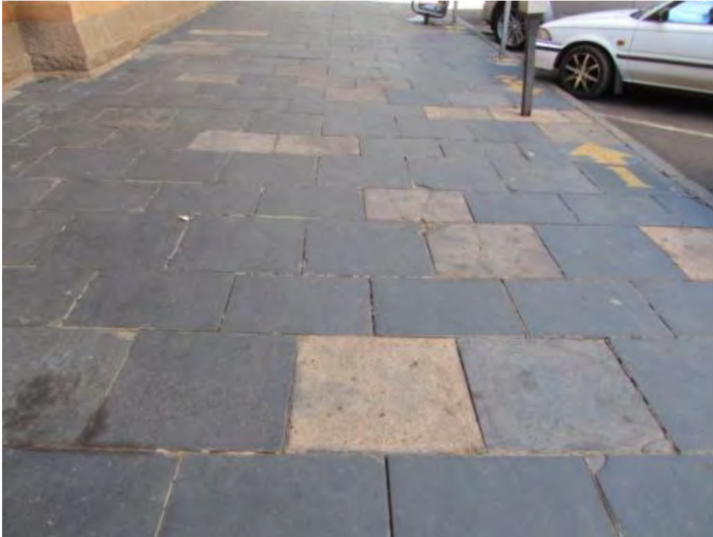
Fig. 54 Historical slate flagstone paving and historical granite kerbing along the central eastern section of Block 3. (Photograph SM Miller 2013)
