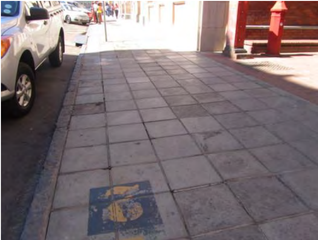
Fig. 28 Modern paving and historical granite kerbing along the south-western section of Block 1. (Photograph SM Miller 2013)
