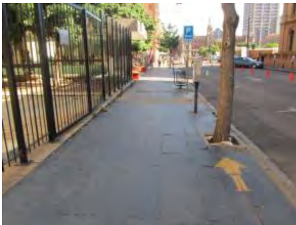
Figs 50 and 51 Historical slate flagstone paving and historical granite kerbing along the central western section of Block 3. (Photograph SM Miller 2013
