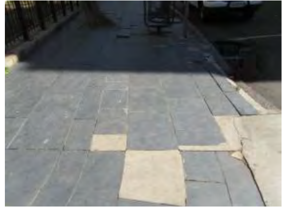
Figs 48 and 49 Historical slate flagstone paving and historical granite kerbing along the south-western section of Block 3. (Photograph SM Miller 2013
