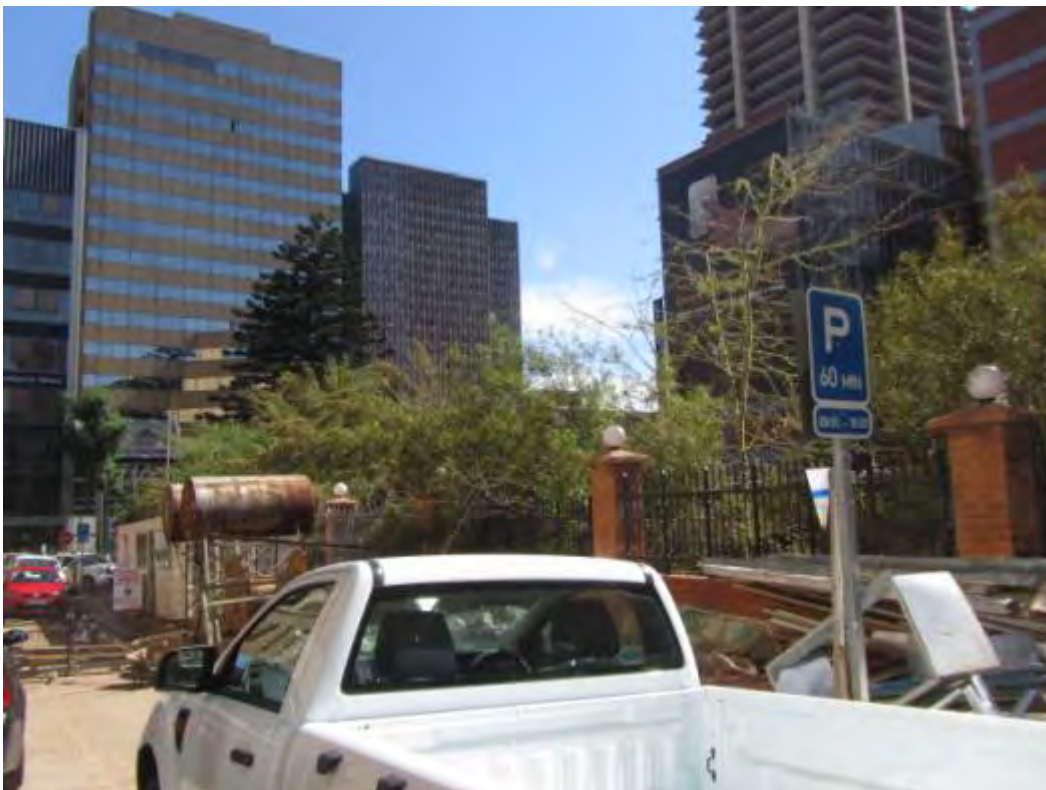
Fig. 39 Mutual Street used as contractor's camp, with a green area in background. (Photograph SM Miller 2013)
