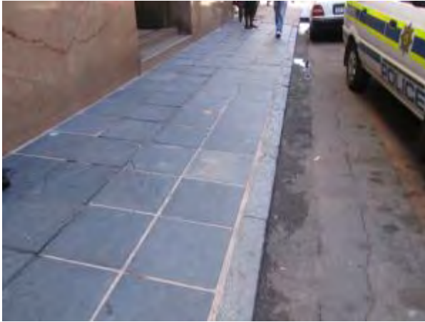
Figs 67 and 68 Historical slate flagstone paving and historical granite kerbing along the north-eastern section of Block 4. (Photograph SM Miller 2013)
