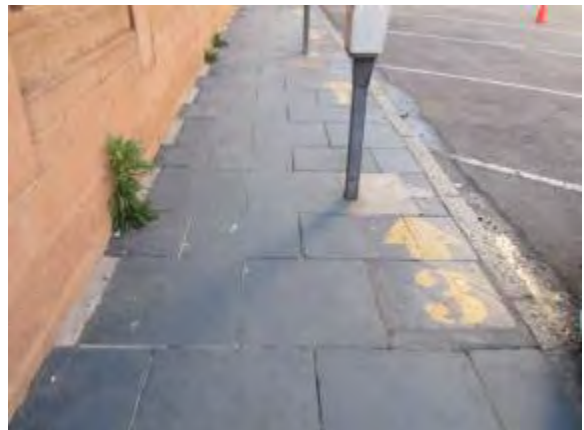
Figs 52 and 53 Historical slate flagstone paving and historical granite kerbing along the north-eastern section of Block 3. (Photograph SM Miller 2013
