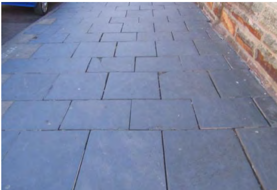
Fig. 22 Historical slate flagstone paving and historical granite kerbing along the south-eastern section of Block 1. It appears as if these flagstones may have been trimmed and re-positioned. (Photograph SM Miller 2013)
