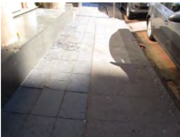
Figs 71 and 72 Historical slate flagstone paving and historical granite kerbing along the north-eastern section of Block 4. (Photograph SM Miller 2013)
