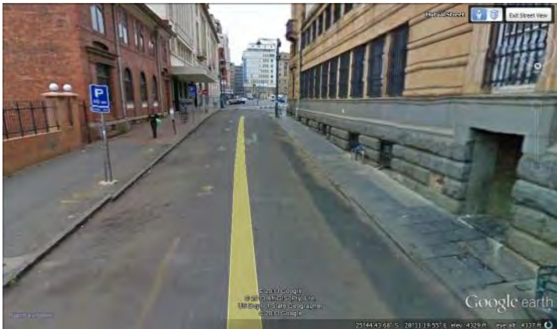
Fig. 45 Image from 2009 showing paving and granite kerbing in Mutual Street. (Google Earth Street View 2009)
