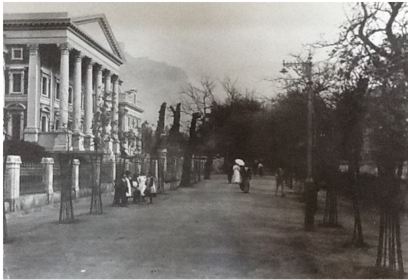
Figure 43: New trees on the foot of Government Avenue. National Archives AG 3322
