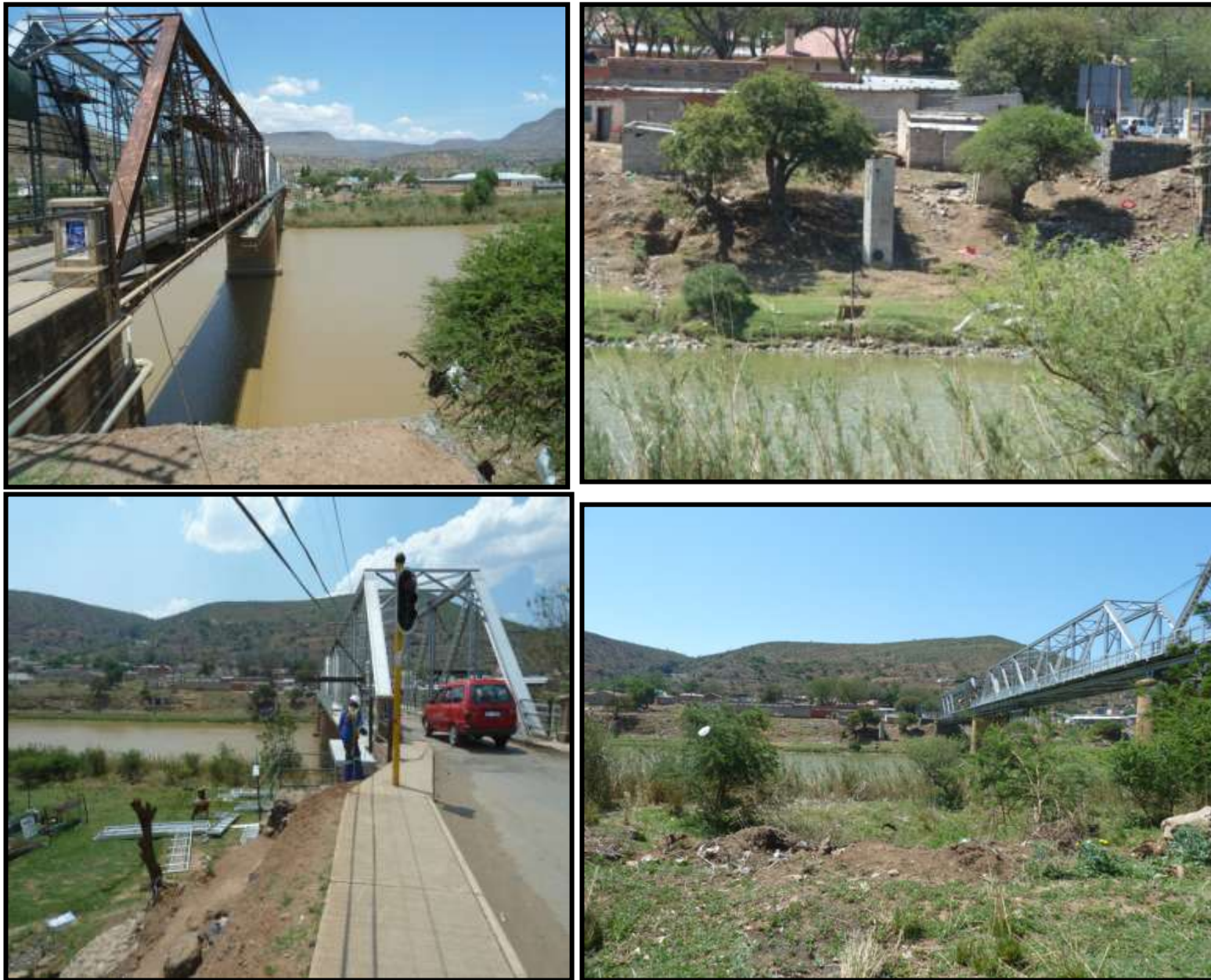
FIG. 8: NORTH AND SOUTH VIEWS OF THE AFFECTED AREA
