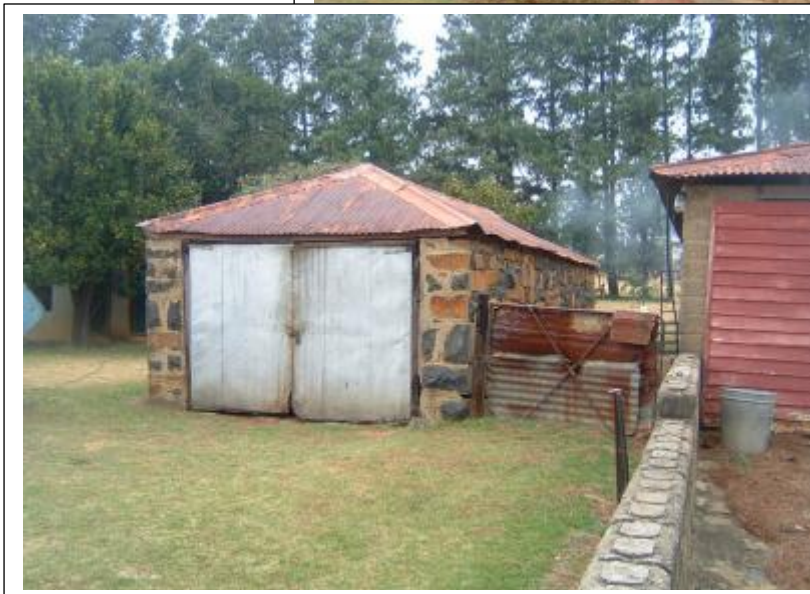
Figures 10, 11 & 12- The main residence (HH02) viewed from the front (above) and the back (centre) and a cattle enclosure (CE02) (below) in Farmstead complex 02. The residence was constructed with sandstone and the wagon shed with dolerite. Both are fitted with corrugated iron roofs.
