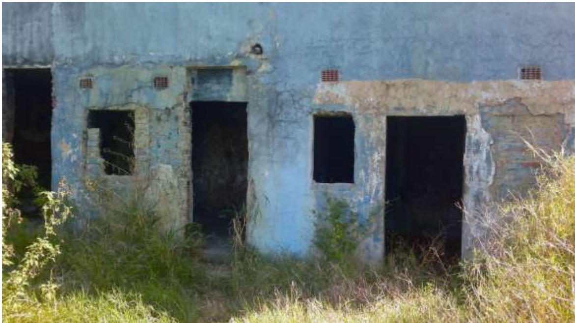
Figure 5: Remains of structure
