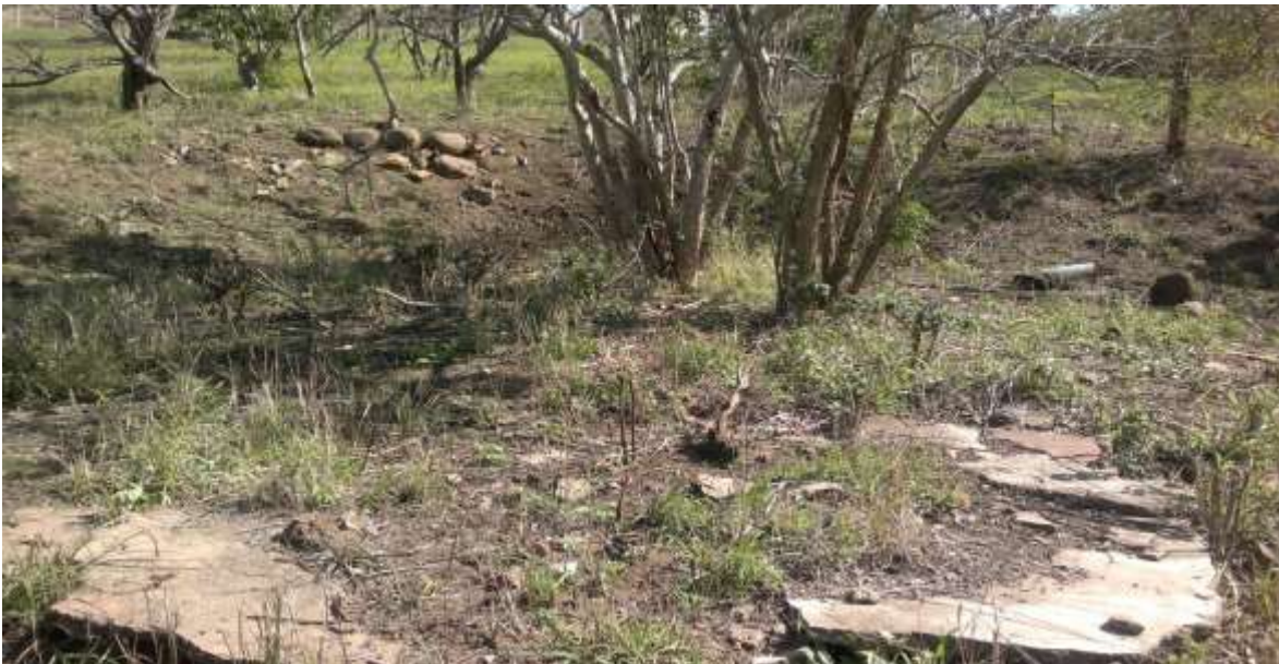
Figure 3: Remains of foundation of demolished structure
