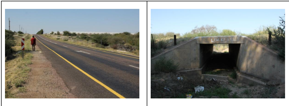
Fig. 28. Views of the bridge.
