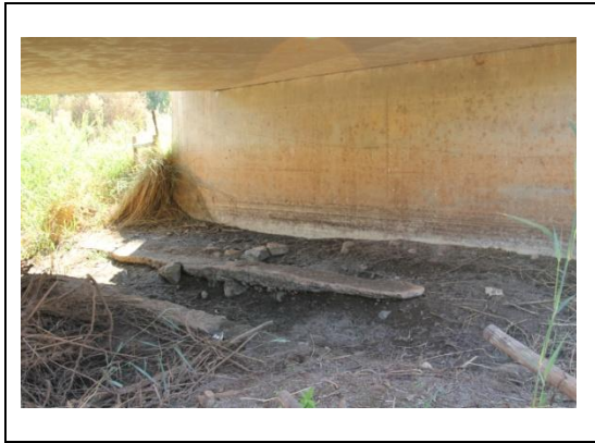
Fig. 10. Old foundation structures
