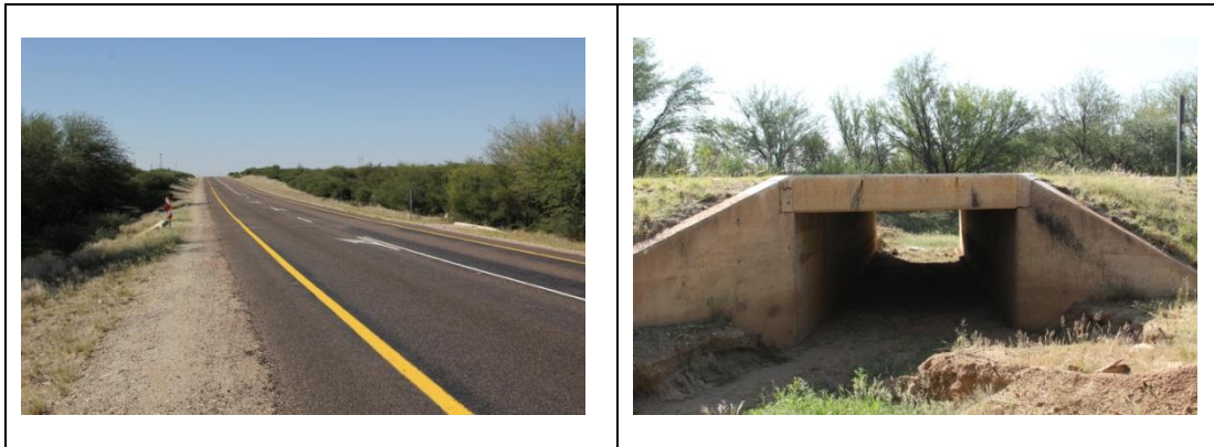
Fig. 25. Views of the bridge.
