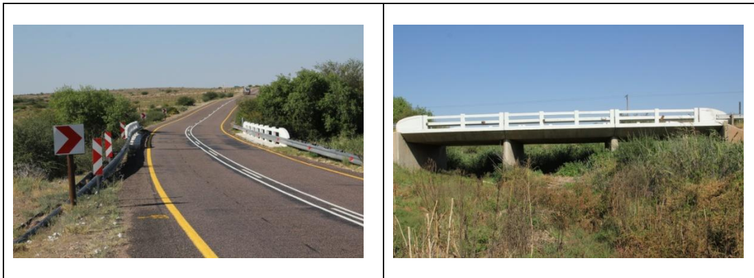
Fig. 5. Views of the bridge.
