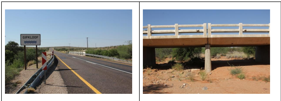
Fig. 12. Views of the bridge.
