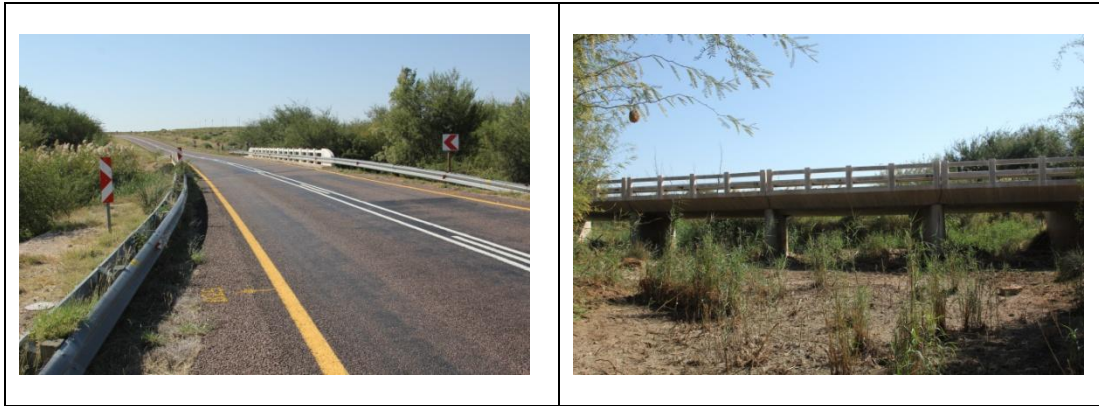
Fig. 8. Views of the bridge.
