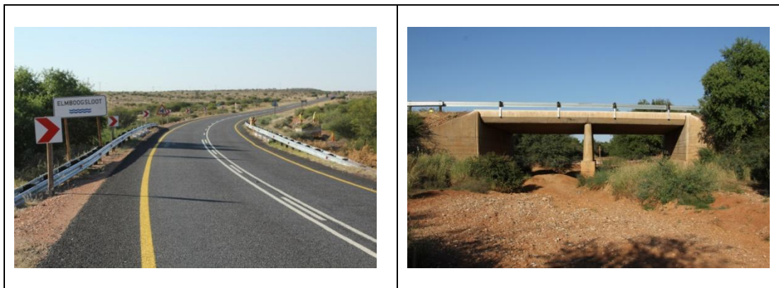
Fig. 2. Views of the bridge.
