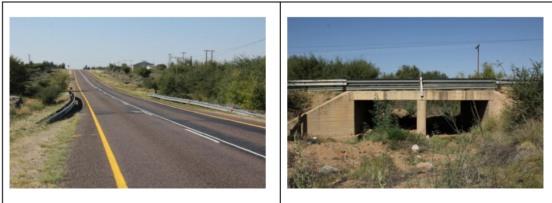
Fig. 22. Views of the bridge.
