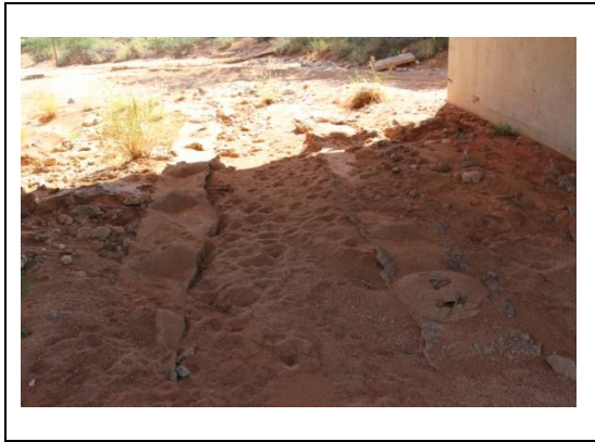
Fig. 14. Old foundation structures
