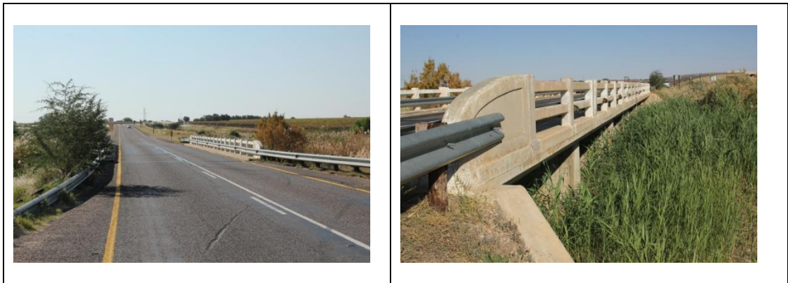
Fig. 16. Views of the bridge.
