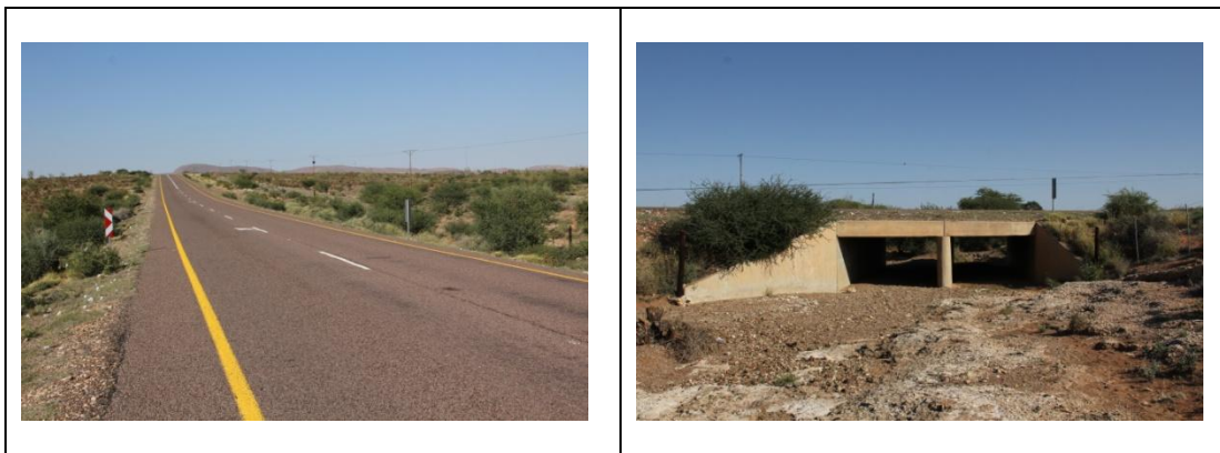
Fig. 19. Views of the bridge.
