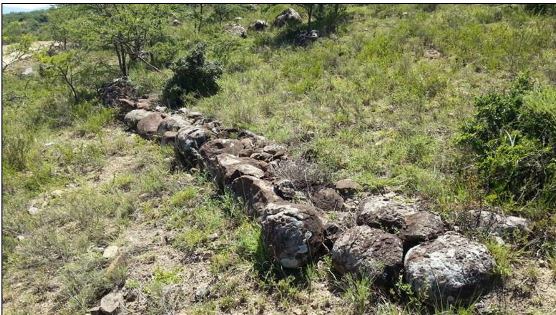
Figure 16: Dry stone walling high and a hill directly adjacent to the exiting reservoir.
