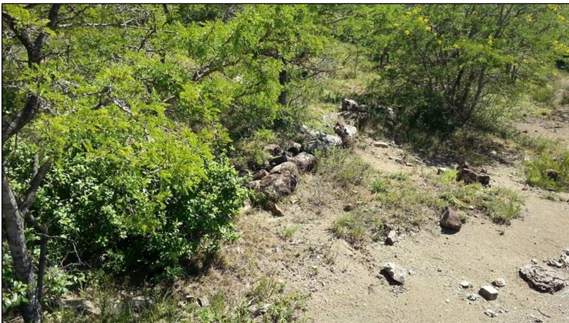
Figure 13: Dry stone walling directly north of the construction site.
