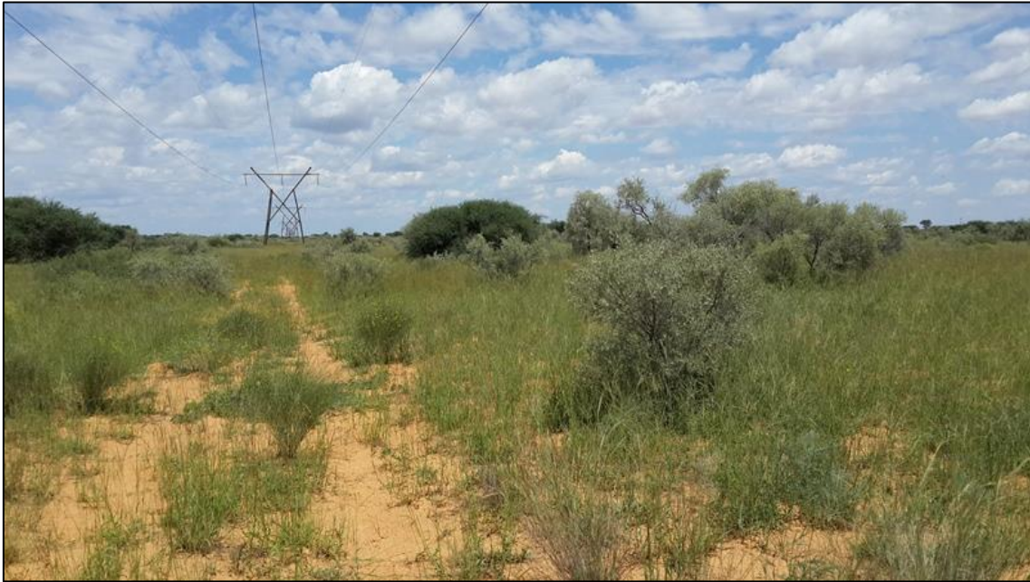
Figure 3-4: View of Corridor 1 along the existing Hotazel - Heuningvlei ESKOM power line near the town of Hotazel.
