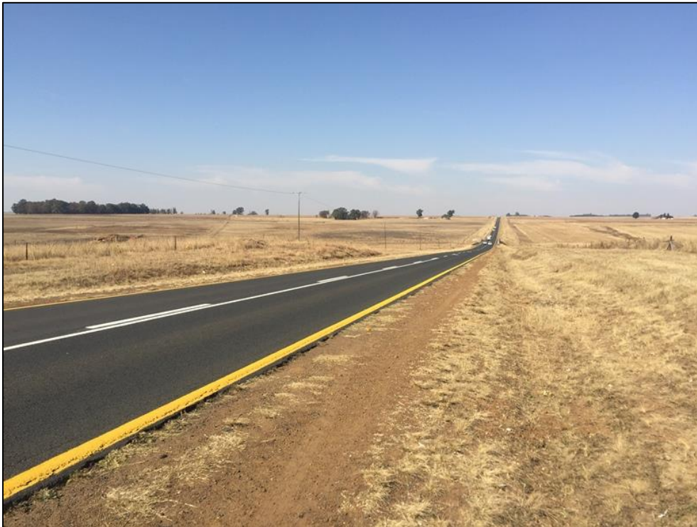
Figure 3-7: View of the N11 route towards Hendrina, subject to the upgrade project.
