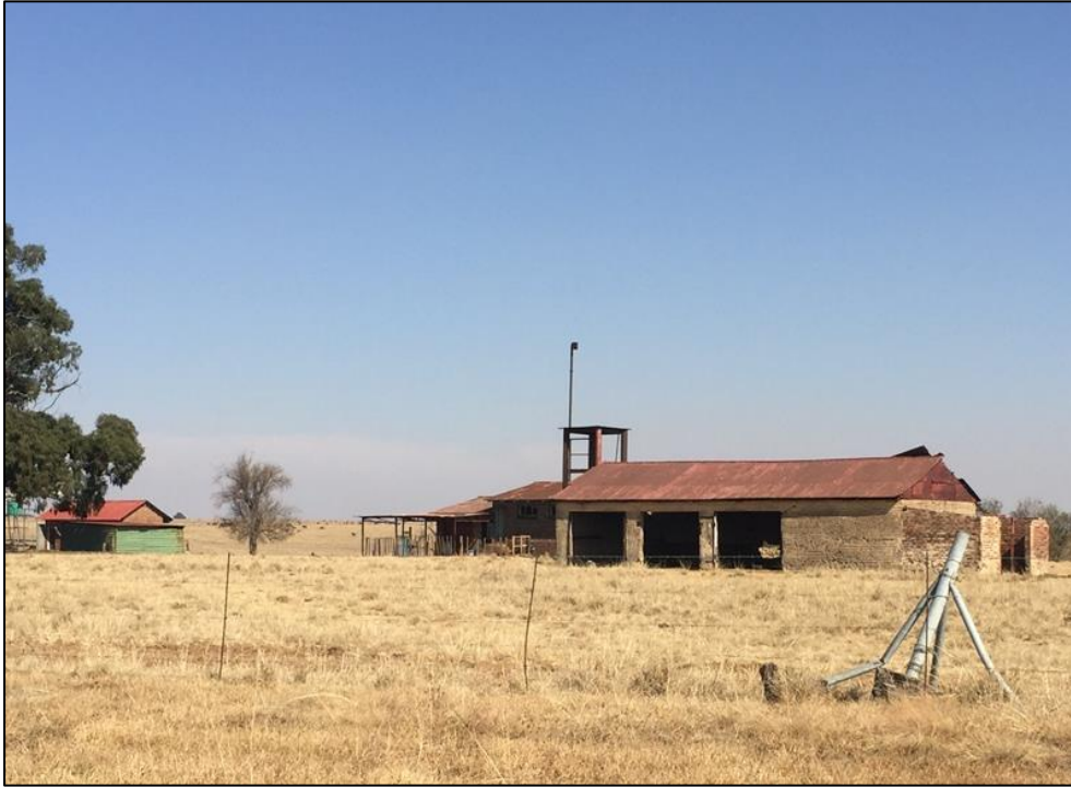
Figure 5-2: Historical Period farming buildings at Site EXIGO-N11UG-HP02.
