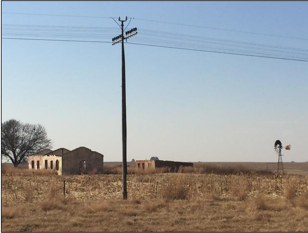
Figure 5-7: Recent period buildings, possibly farm workers houses at Site EXIGO-N11UG-FT02.
