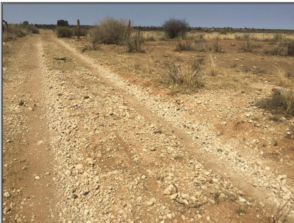
Figure 18: View of a decomposing calcrete horizon along the proposed access road at Site Exigo-WE681-SA03.
