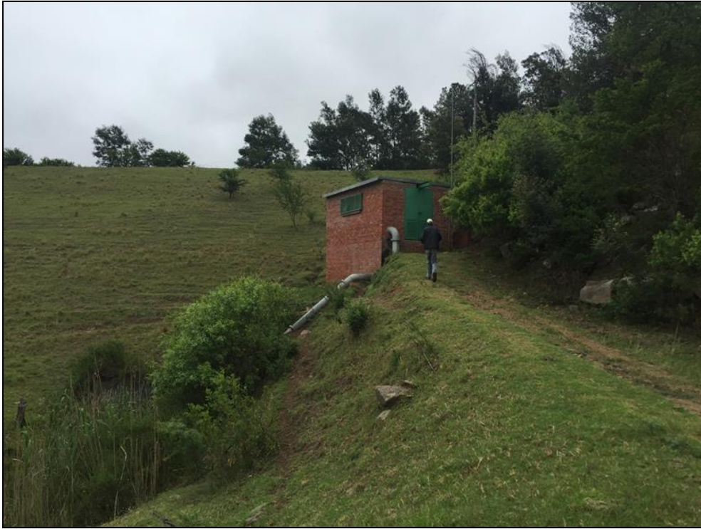
Figure 3-2: View of a small pump station at the Sam Meyer Dam wall in the proposed Cathcart Bulk Water and Sewer Line Project Area.
