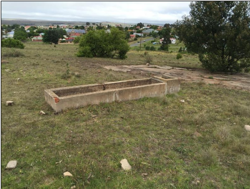
Figure 5-5: A concrete cattle drinking trough at site EXIGO-CWS-FT01.
