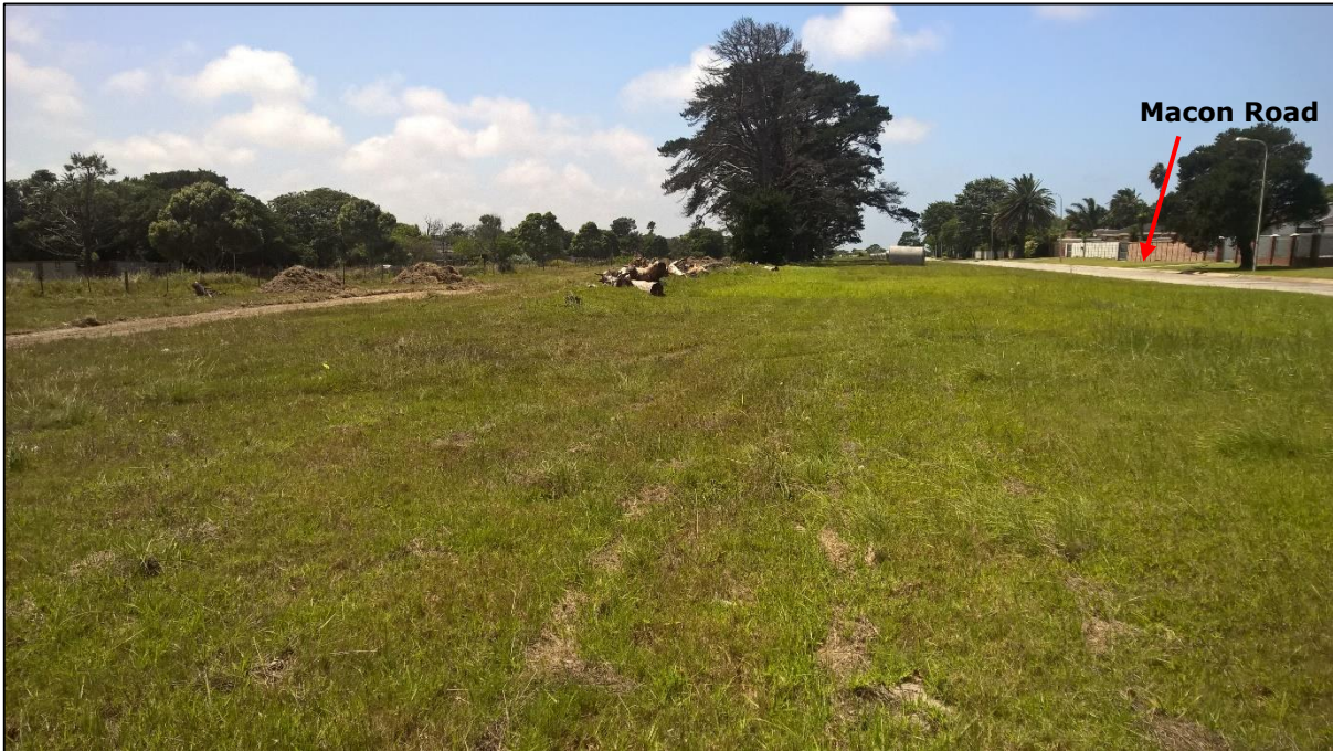
Figure 9. View from the Lorraine substation facing east showing Macon Road, the circular concrete structures, new/upgraded gravel road and the railway line.
