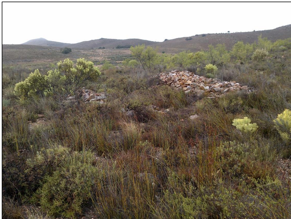
Figure 16. Example of stone packed erosion prevention walls.
