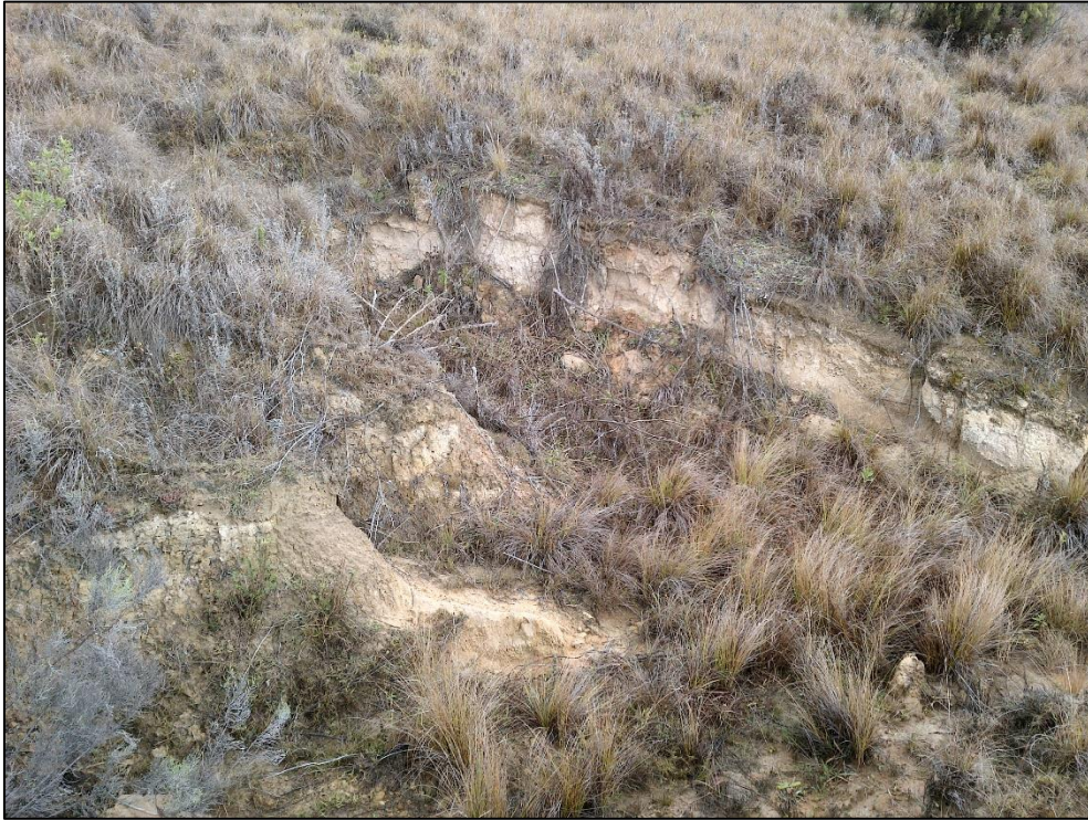
Figure 12. Example of surface eroded area.
