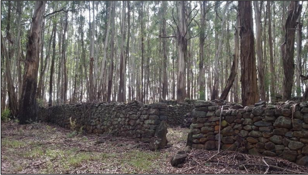
Figure 5-1: Extensive stone walling and enclosures at Site EXIGO-RK133JT-HP01. Note entrance in the structure.
