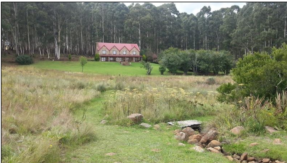
Figure 3-6: View of the current Roodekrans farm house. Note the Eucalyptus forest east of the house.
