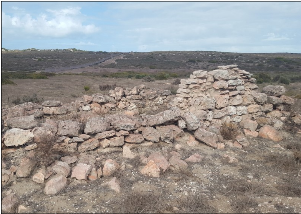
Figure 5-2: A large rectangular stone structure at Site EXIGO-VTP-HP01. Note mortar fill in wall construction.
