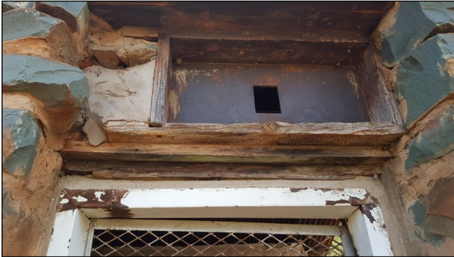
Figure 5-31: View of a corner loophole in the exterior of the blockhouse.
