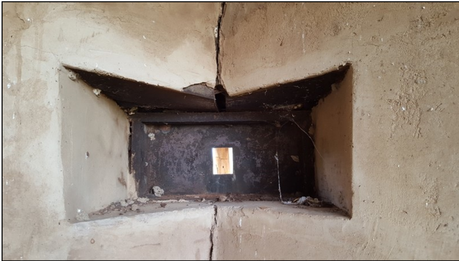
Figure 5-28: View of a corner loophole in the interior of the blockhouses.
