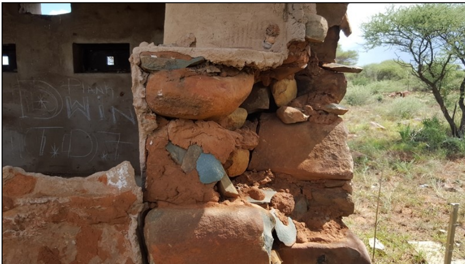
Figure 5-28: View of a corner loophole in the interior of the blockhouses.
