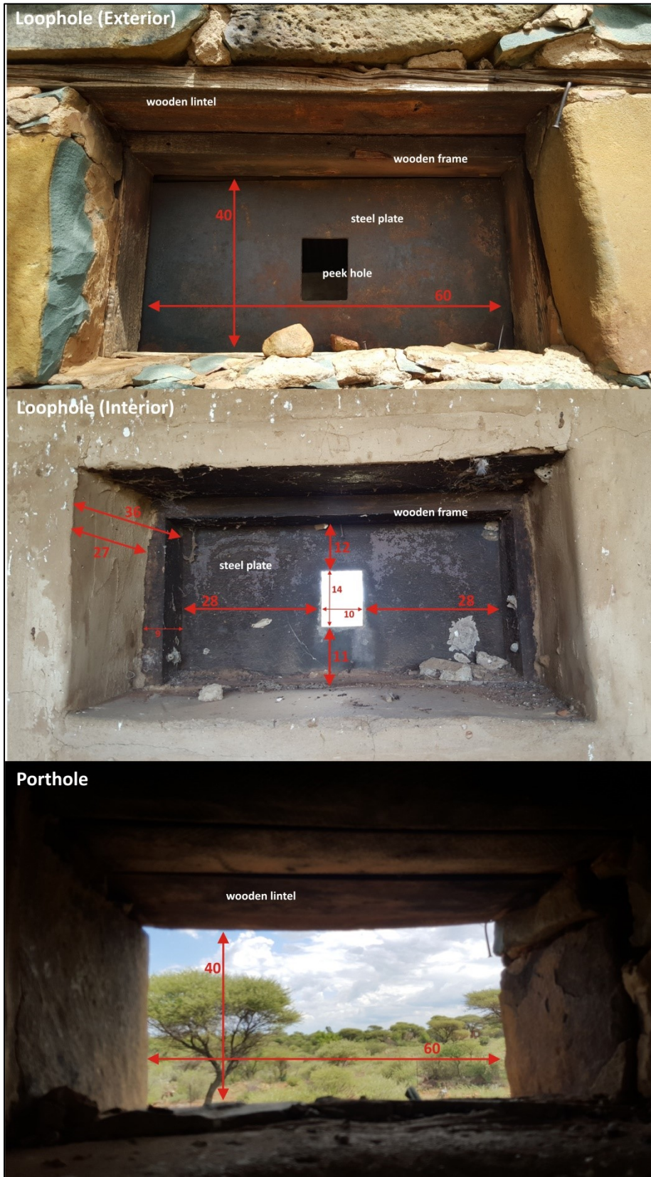
Figure 5-41: Schematic representations of loophole and porthole dimensions.
