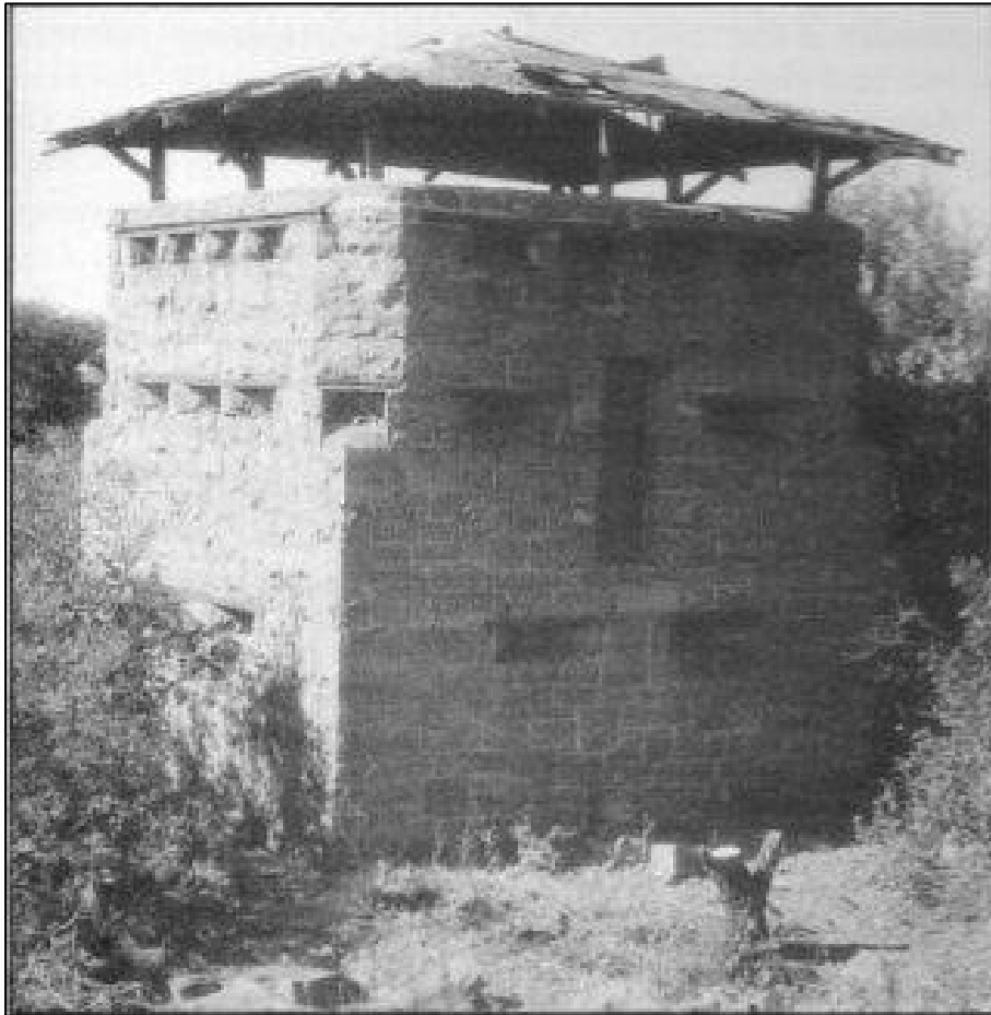
Figure 5-19: The old Warrenton Railway Bridge Blockhouse, now dilapidated.
