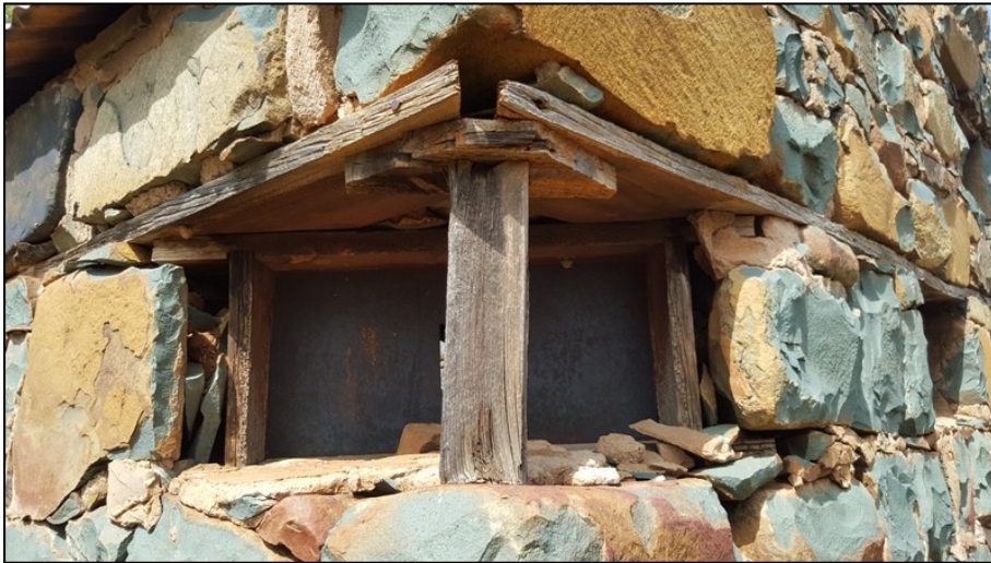
Figure 5-31: View of a corner loophole in the exterior of the blockhouse.
