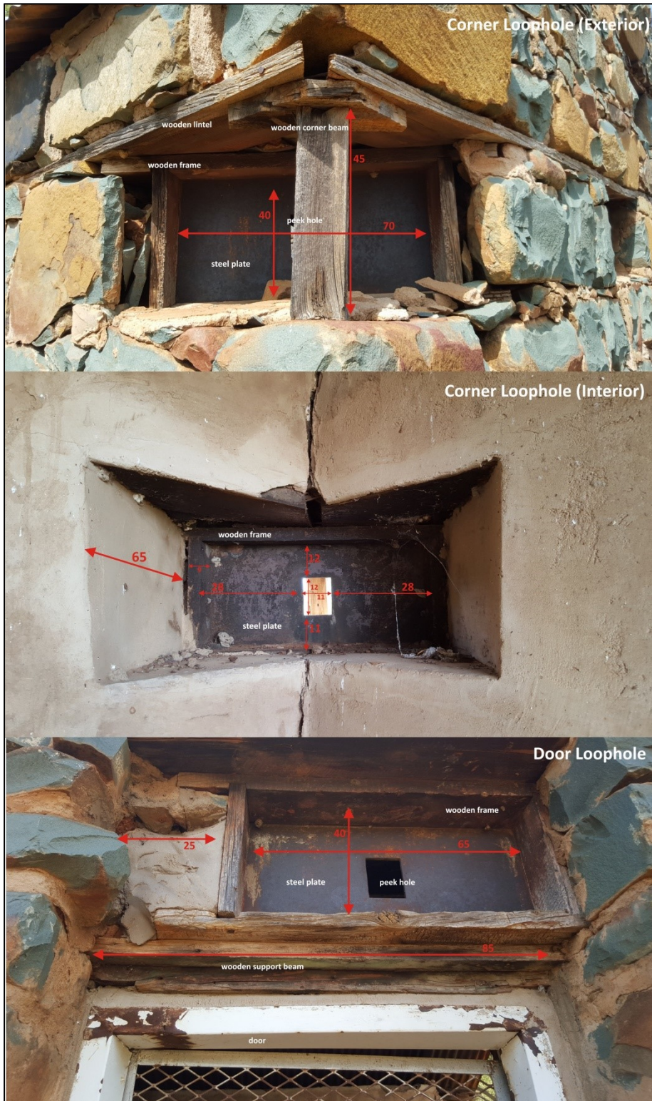
Figure 5-42: Schematic representations of loophole dimensions.
