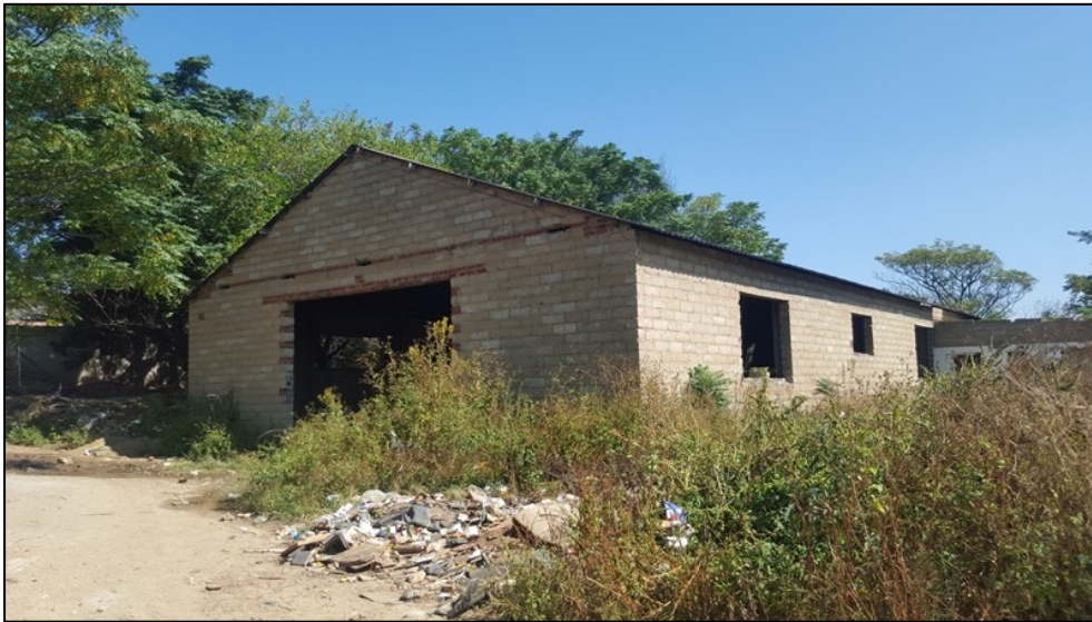
Figure 5-19: A partially constructed shed building Site EXIGO-ZTE-CP08.
