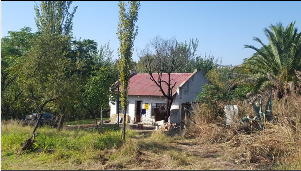
Figure 5-1: A small Historical Period house at Site EXIGO-ZTE-HP01.
