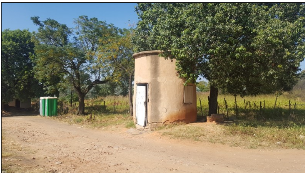
Figure 5-5: A cylindrical structure, possibly a grain storage container at Site EXIGO-ZTE-HP02.
