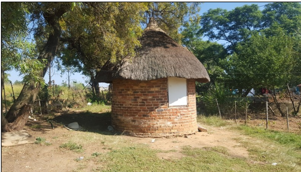
Figure 5-4: A small rondavel at the compound demarcated as Site EXIGO-ZTE-HP02.
