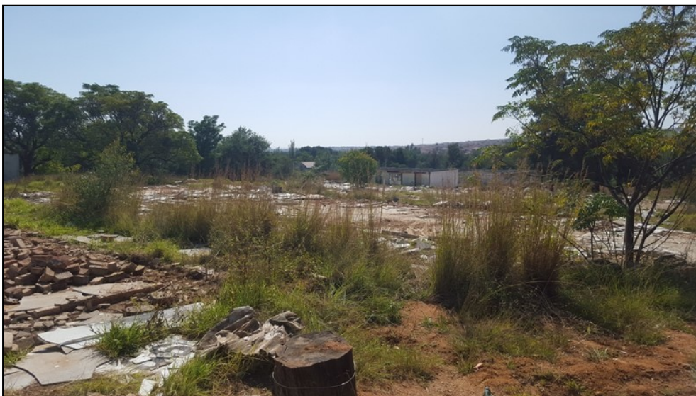
Figure 3-7: Large foundations structural remains of a factory in a central part of the project area.
