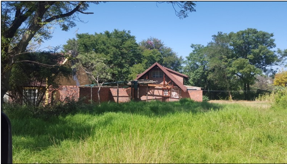
Figure 5-13: A modern Contemporary Period residence at Site EXIGO-ZTE-CP03.
