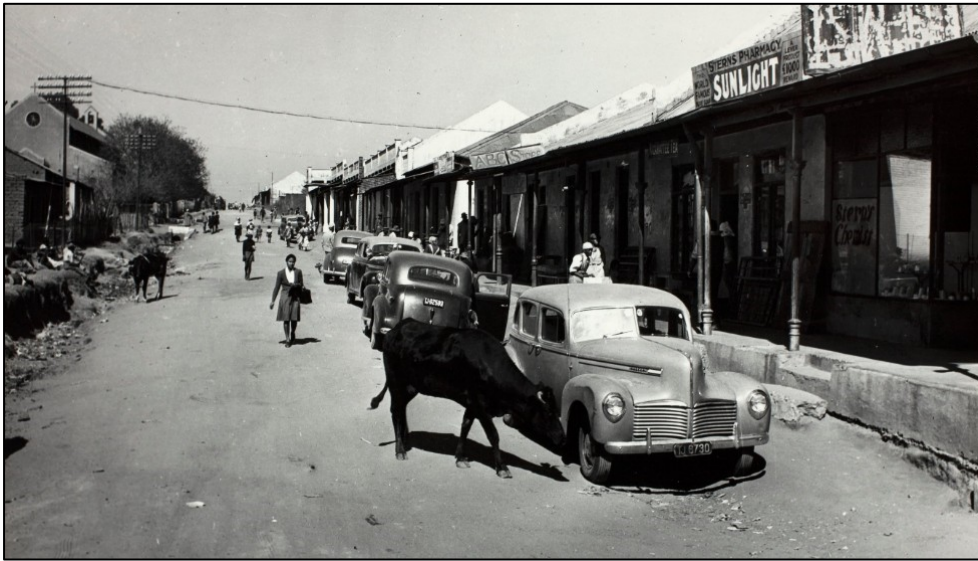
Figure 4-1: View of a street in the Zandspruit township in the 1970's.
