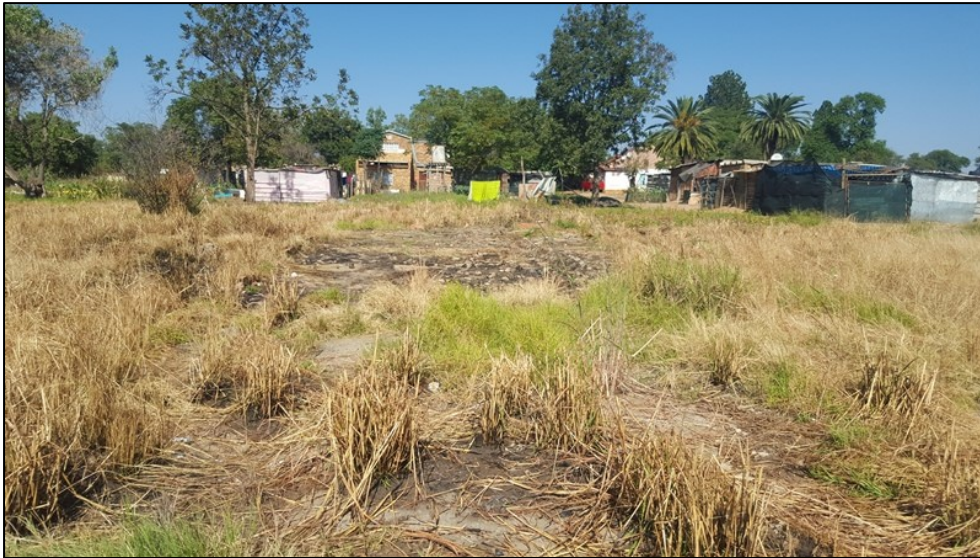
Figure 5-12: Foundation structures at Site EXIGO-ZTE-CP02.
