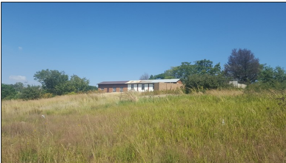
Figure 5-18: A factory building at EXIGO-ZTE-CP07.
