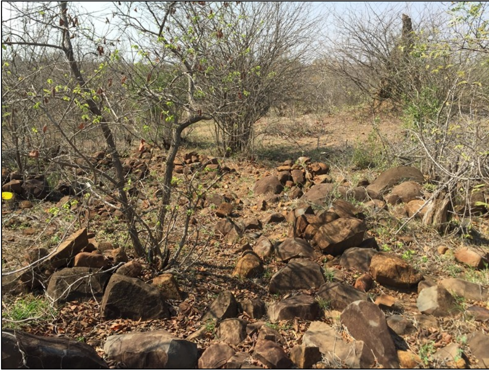
Figure 5-7: Collapsed stone walling at Site EXIGO-BSP-IA03.
