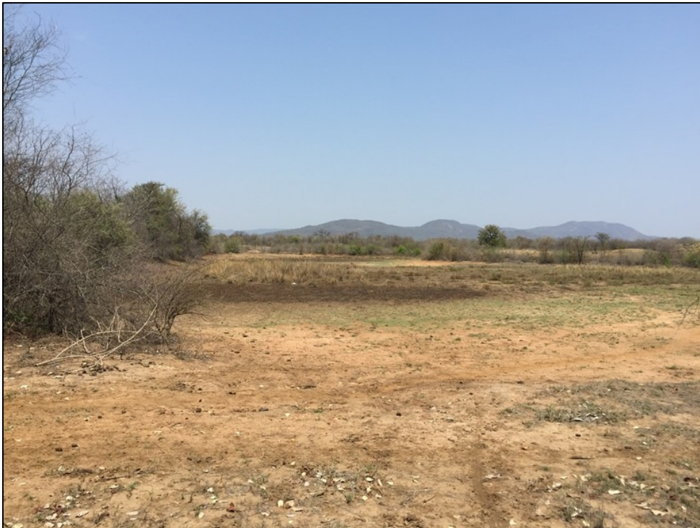
Figure 3-11: View of a small dam in the study area.
