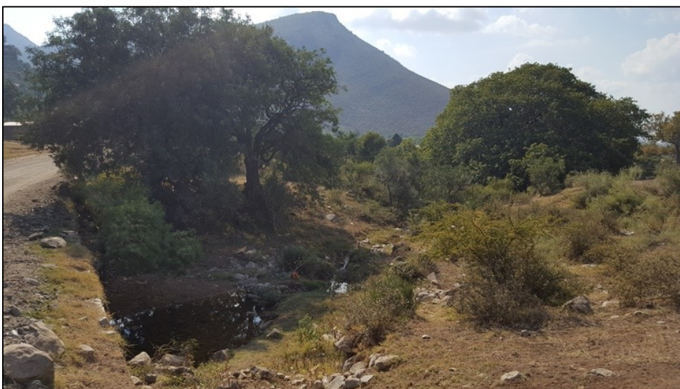
Figure 3-8: View of a drainage line where the alignment deviates from the existing road at Makgake.
