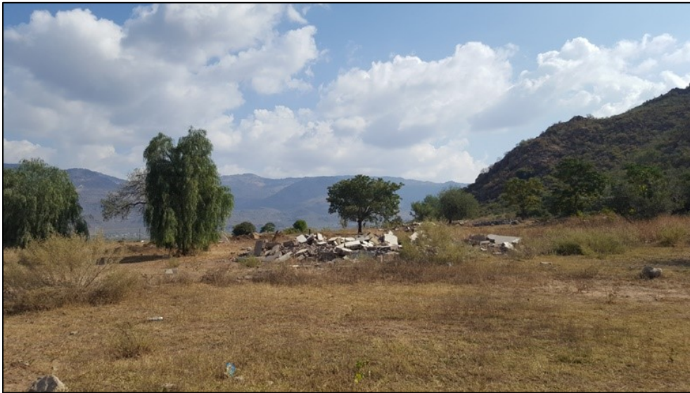
Figure 3-6: Demolished brick buildings along the road alignment near Ga-Mashabela.
