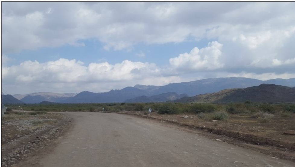
Figure 3-2: View of the current road to be upgraded, approaching the village of Modlimolle.
