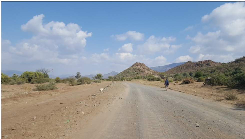
Figure 3-7: General surroundings in the project area between Ga-Mashabela and Makgake.
