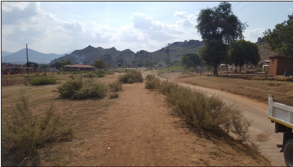
Figure 3-9: View of the existing road to be upgraded approaching the village of Magakala and the north-western offset of the upgrade alignment.
