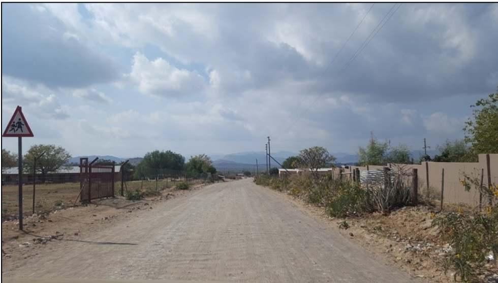
Figure 3-5: A section of the road to be upgraded through the village of Ga-Montane.
