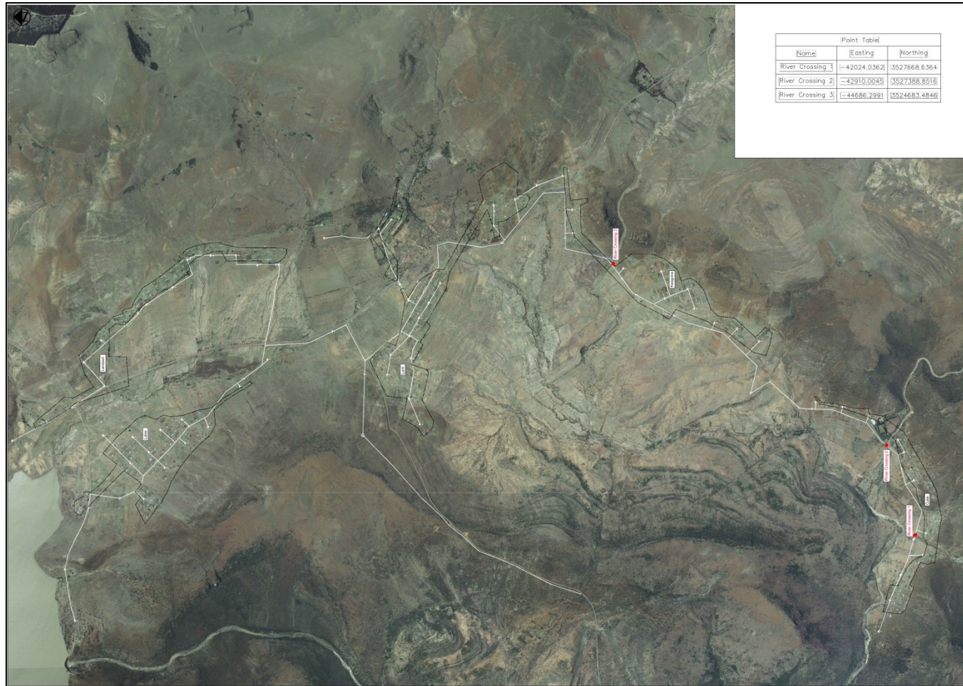
Figure 1-1: Aerial image indicating infrastructure components subject to the Cluster 2 RS5-3 Water Supply Upgrade Project.
