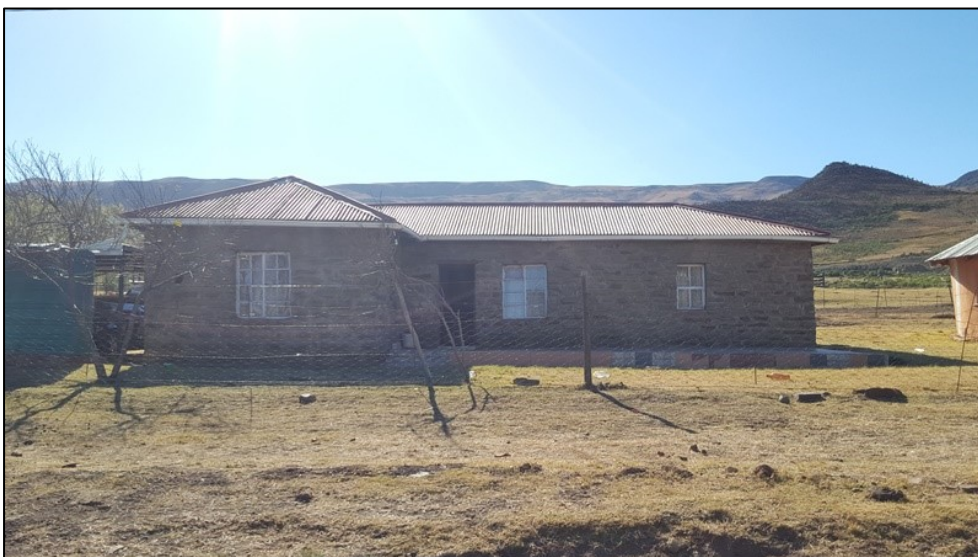
Figure 5-16: A stone house probably dating to Colonial Times at Site EXIGO-CL2-HP06.
