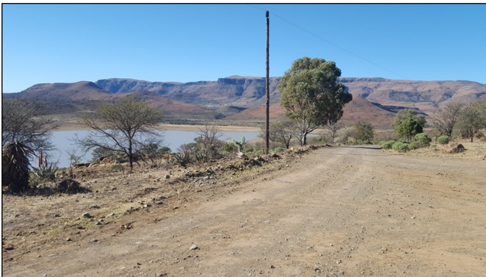
Figure 3-1: View of the southern banks of the Lubisi dam.
