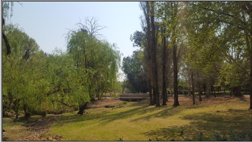
Figure 5: The Hartebeest Spruit and "Culvert A" in the LC de Villiers Culverts Project area.
