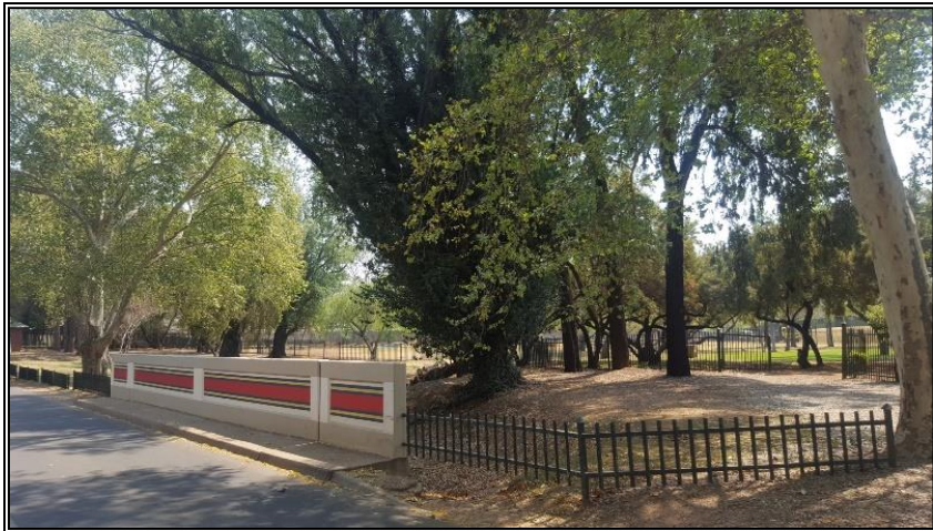
Figure 6: View of a concrete bridge over "Culvert A" and the Hartebeest Spruit.
