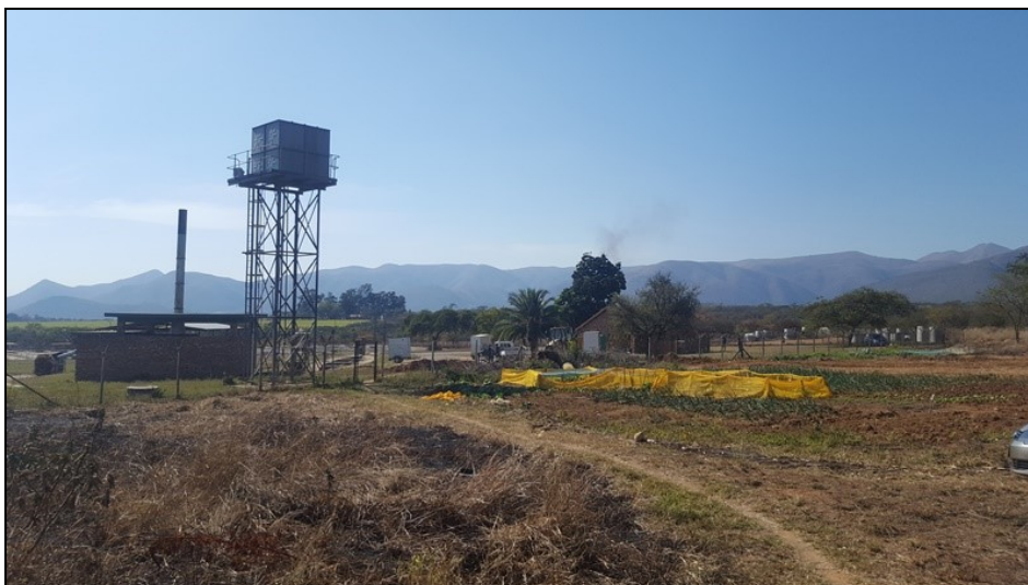
Figure 3-2: View of the existing water treatment works along the east of the study area (July 2016).
