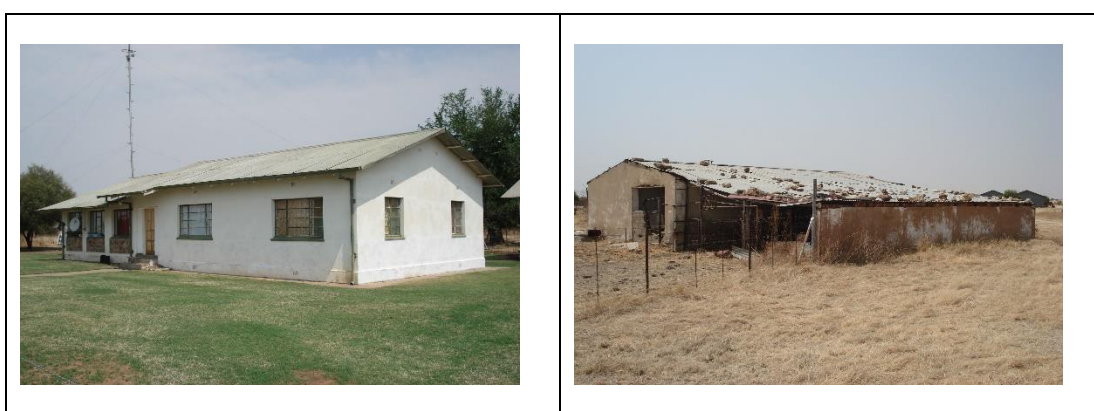
Fig. 5. Existing structures (main house and barn) on the farm.
