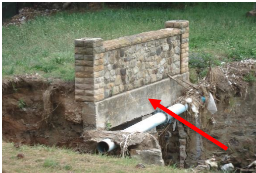
Concrete bridge deck
