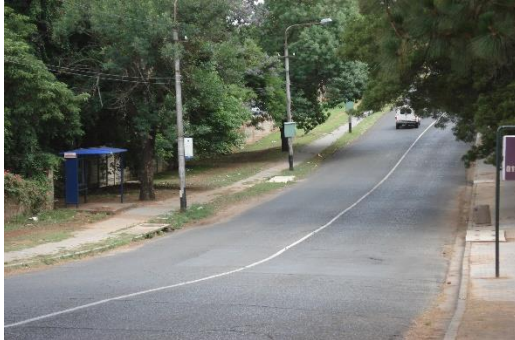
Current approach road
