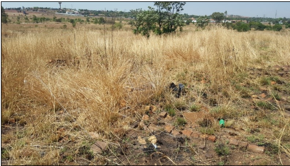
Figure 3-3: A brick foundation visible on the surface at Site Exigo MDW-HP01 Feature 1.
