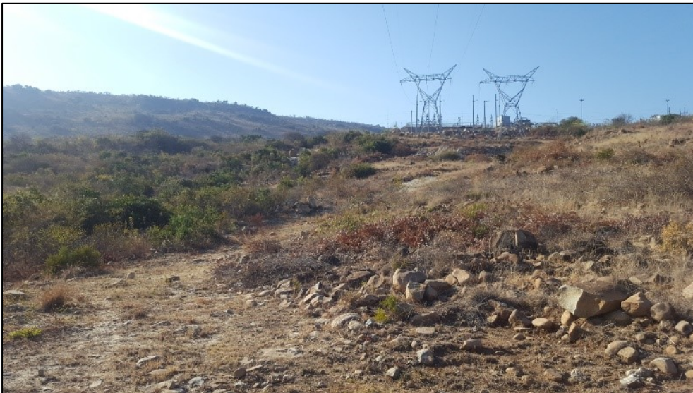
Figure 3-10: View of a power line aligning north of the site proposed for the northern pollution control dam.
