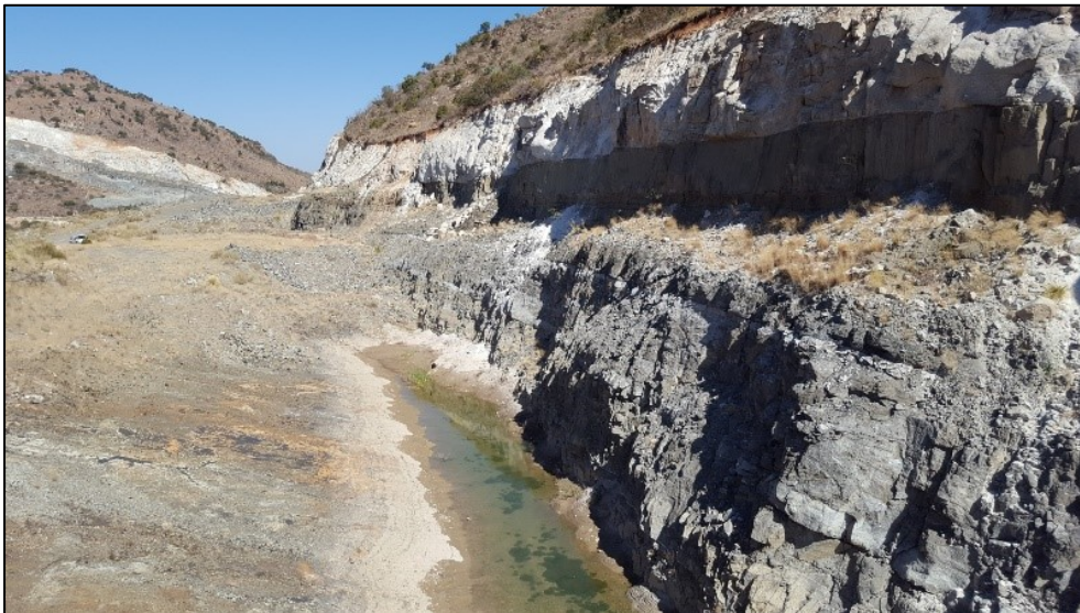
Figure 3-7: A decommissioned opencast mining quarry on Hill 2 at the site of the proposed central pollution control dam.
