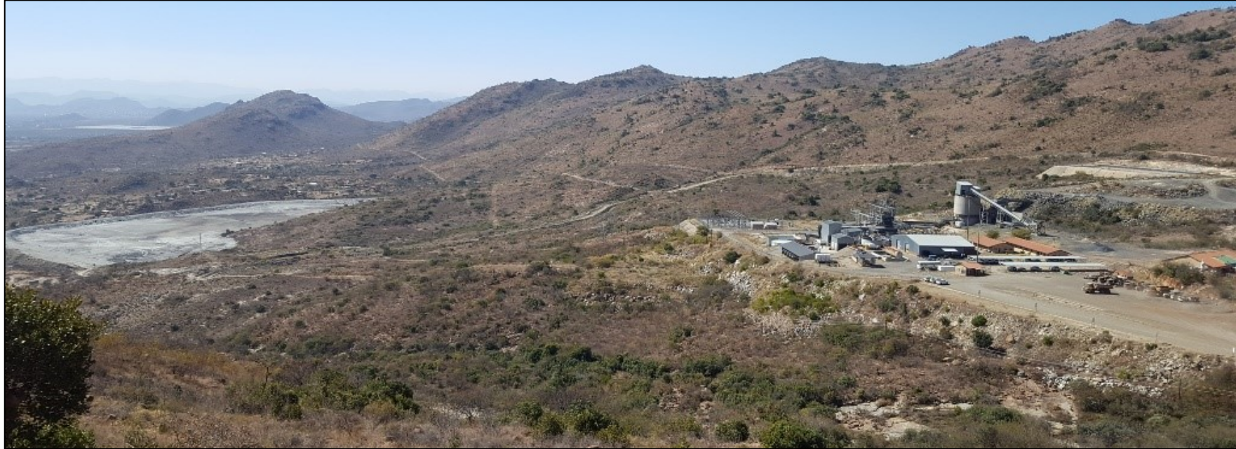
Figure 2-3: View of the Smokey Hills Mine, looking north. The mine plant and offices are visible to the right and the tailings dam occurs to the west on the left.
