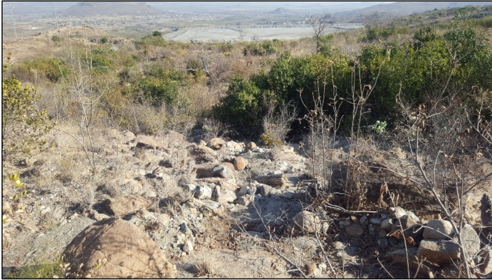
Figure 3-12: Surface rock and degraded calcrete in the proposed northern pollution control dam footprint.
