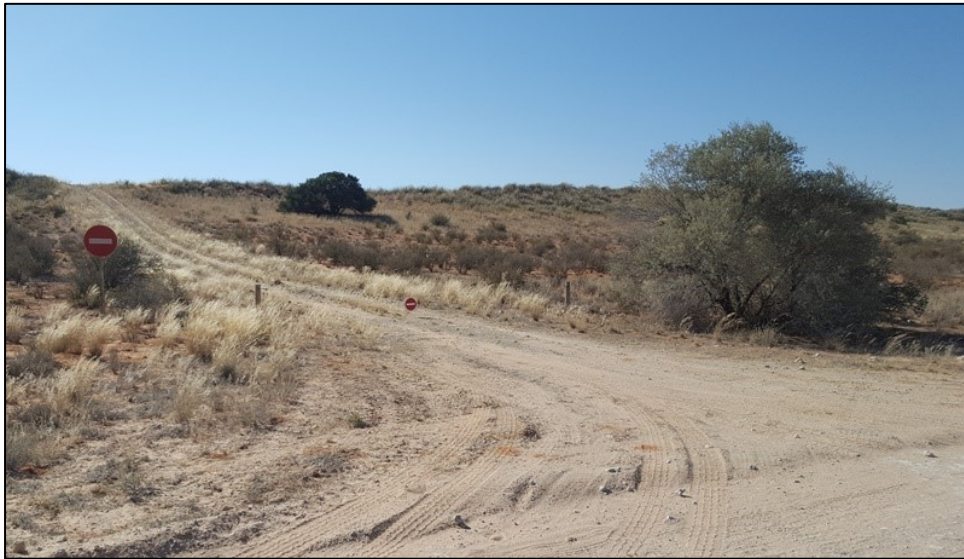
Figure 3-11: The existing service road to the project site - to be upgraded.
