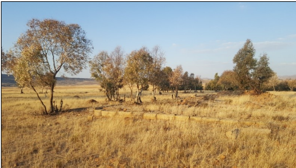
Figure 5-3: The ruined foundation remains of a Historical Period dwelling east of the project area.
