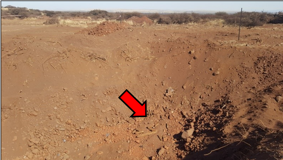
Figure 4-10: View of the excavation trench where human remains were exposed (red arrow).
