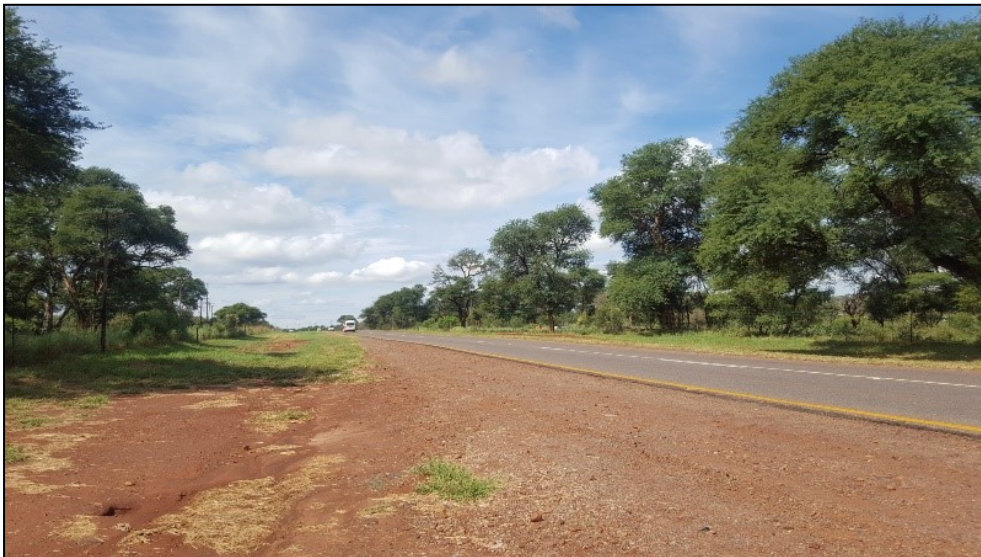
Figure 3-5: View of the R510 road in a central portion of the upgrade project area.
