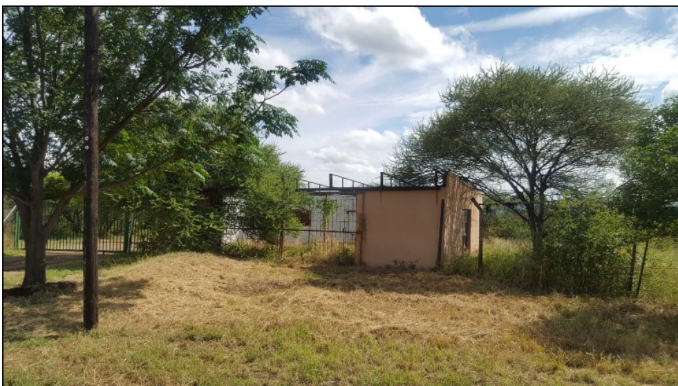
Figure 3-3: A disused farm stall along the R510 road.
