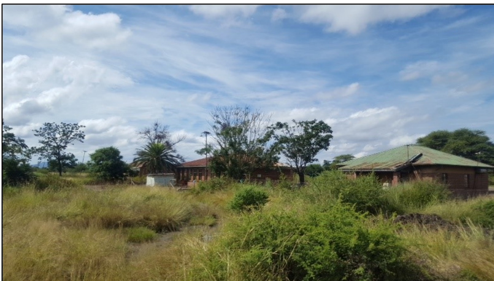
Figure 5-2: View of red brick structures, possibly railway station buildings at Site EXIGO-R510UG-HP01.
