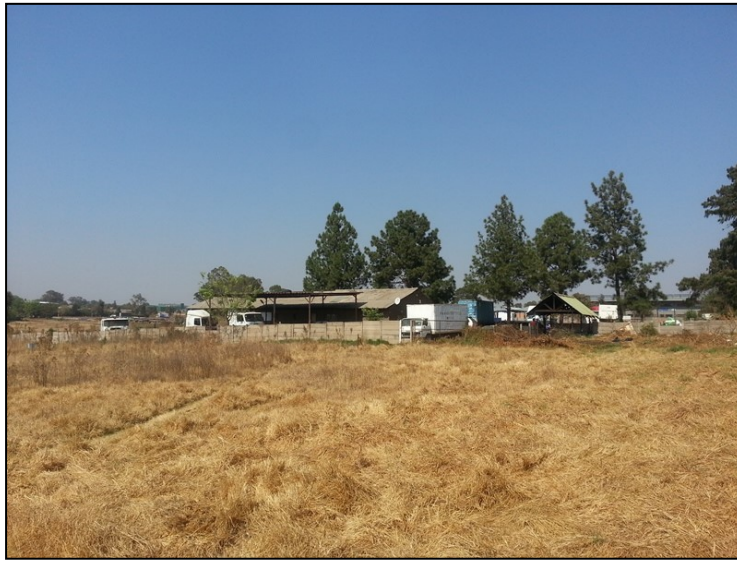
Figure 3-6: The truck depot in the centre of the project area.
