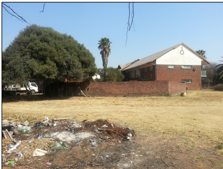
Figure 5-5: View of a multi-storey contemporary period residence at Site EXIGO-PWD-FT03.
