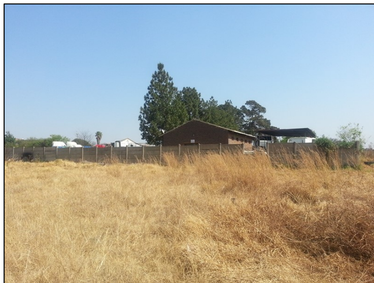
Figure 3-8: The building for the truck depot in the project area.
