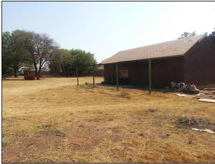
Figure 5-6: A small contemporary period outbuilding within the compound at Site EXIGO-PWD-FT03.
