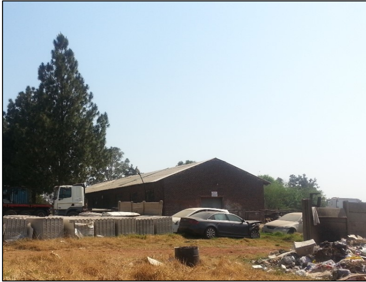
Figure 5-8: View of the buildings at the truck depot in the project area at Site EXIGO-PWD-FT04.
