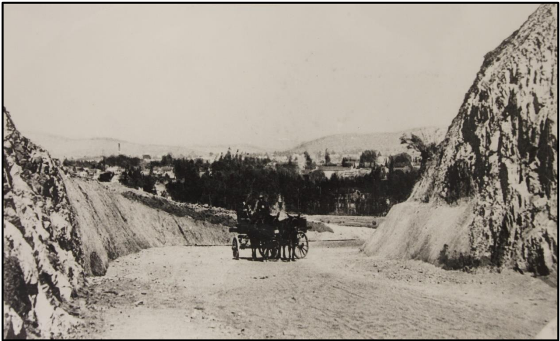
Figure 10. Contemporaneous photograph of Eloff Cutting, looking south.
