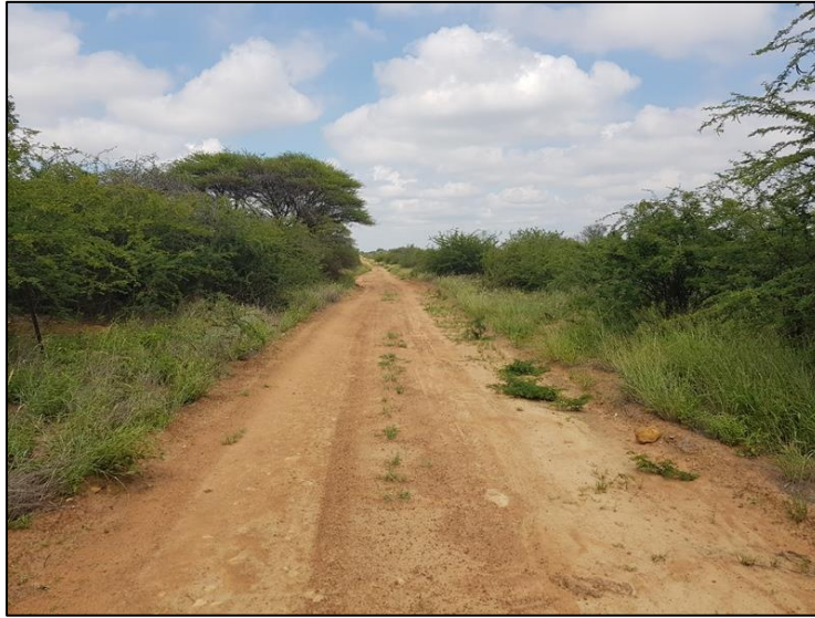
Figure 3-6: The Transnet service road along the proposed railway loop alignment, looking south.
