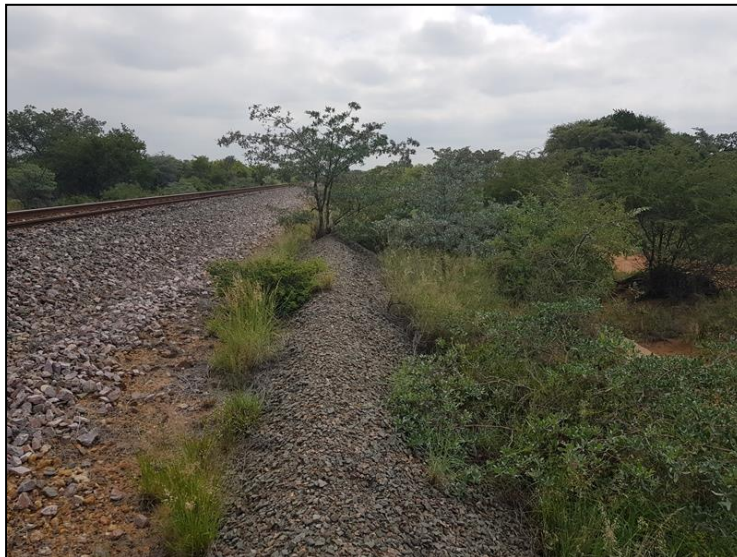
Figure 3-4: View of the current railway line. The proposed railway loop will be constructed directly right of this line.
