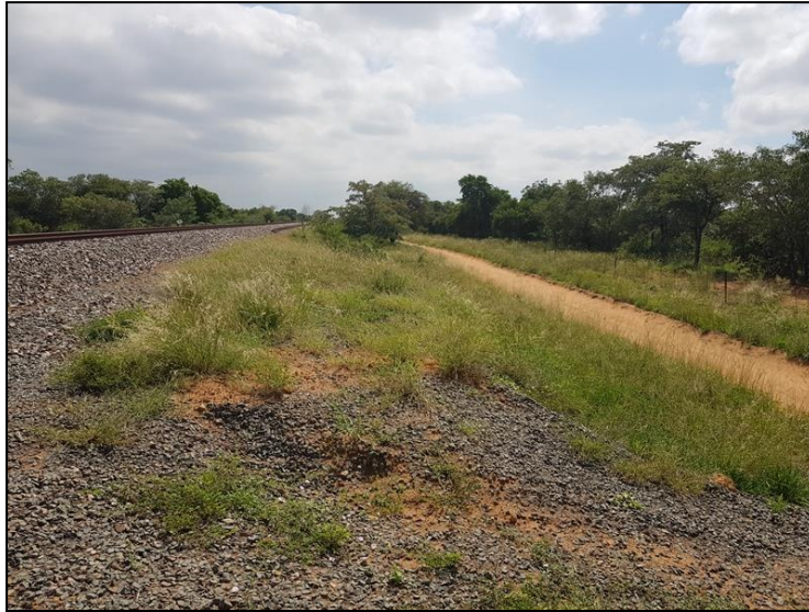
Figure 3-1: View of the project area at the southern offset of the proposed railway loop alignment.
