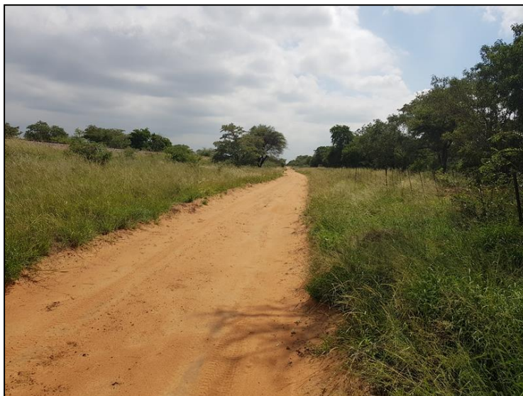
Figure 3-2: The Transnet service road along the proposed railway loop alignment.
