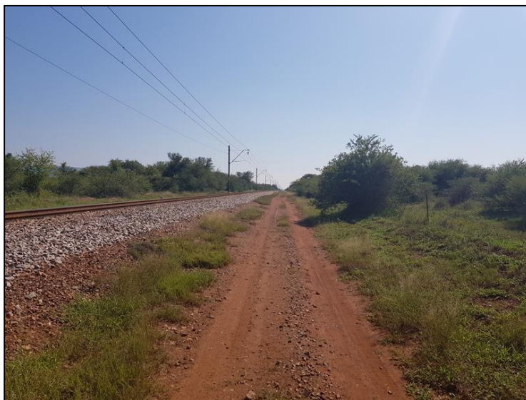
Figure 3-4: View of the railway loop alignment area.
