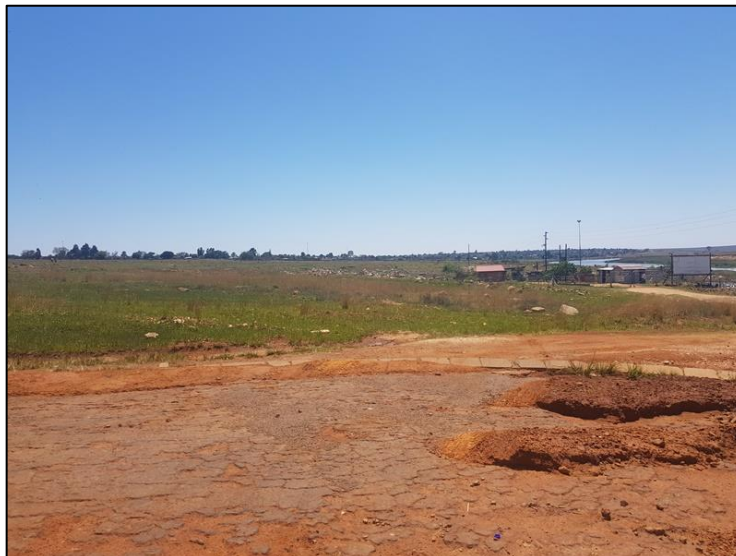
Figure 3-15: View of the existing Waste Water Treatment Works to the south-east of the project area.
