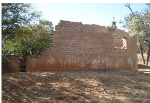
Old nursery facility
